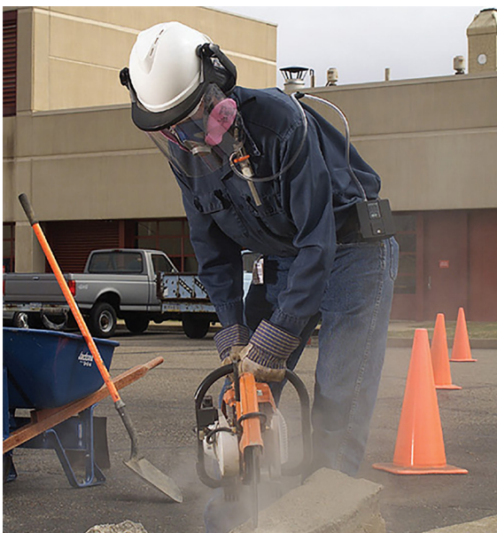
Figure 2: Worker with cutoff saw and personal air monitoring equipment.
