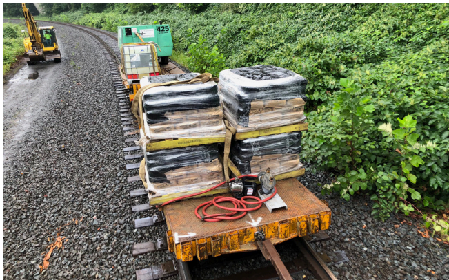
Emergency Tunnel Repairs
