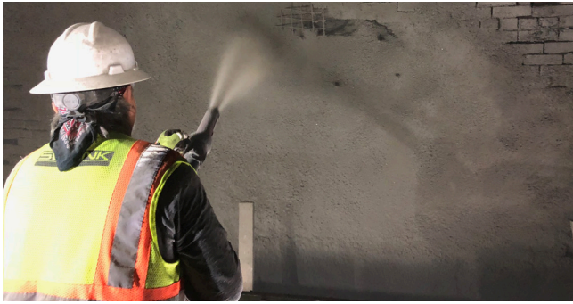
Railroad Tunnel Shotcrete Repair
