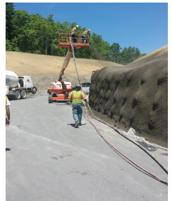
Newburgh Water Tunnel Bypass Project; a rock stabilization job. The production line for 5000 PSI wet-mix ran up to 60' above the ground, holding back the earth for the new access road for an aqueduct tunnel providing potable water to the residents of New York City.
