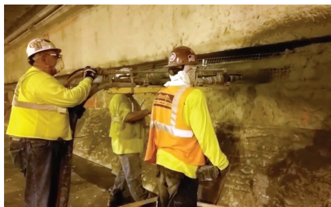
Nozzleman innovation for fireline encapsulation, 5-feet off the ground, at the Queens Midtown Tunnel. (2019 Outstanding Shotcrete Award)
