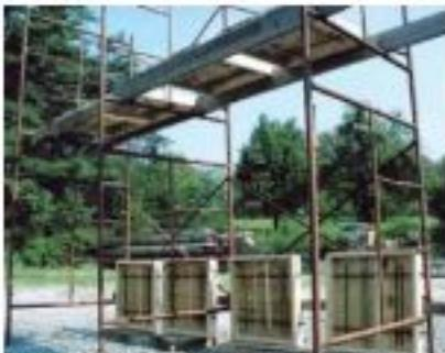
The scaffolding set up for both the overhead and vertical panels
