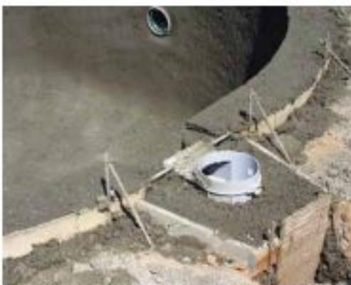
*Typical batter board form work around a swimming pool that sets the shape, elevation, and dimensions*
