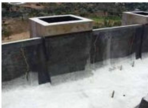
Finishing edge weir wall where shrinkage cracks reflected through water line tile. Repair was by epoxy injection.
