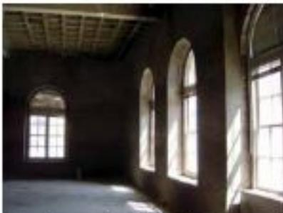
*Internal corner with reinforced shotcrete around arched windows*
