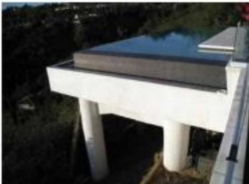
*Pier-supported, out-of-grade swimming pool required complicated false work during construction*
