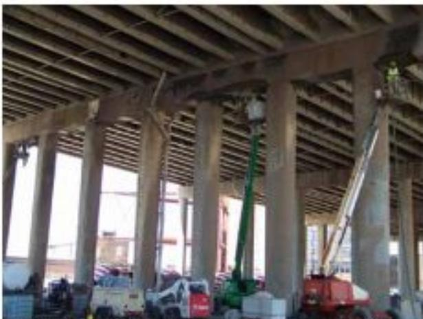
All shotcrete work was done from the ground and pumped upward to the nozzle
