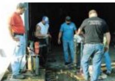
*The core drilling of the shotcrete panels the day after gunning*
