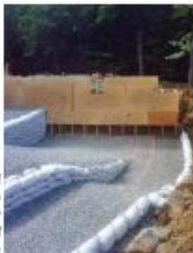
Stone-filled bags used to create floor profiles of pool and catch basin
