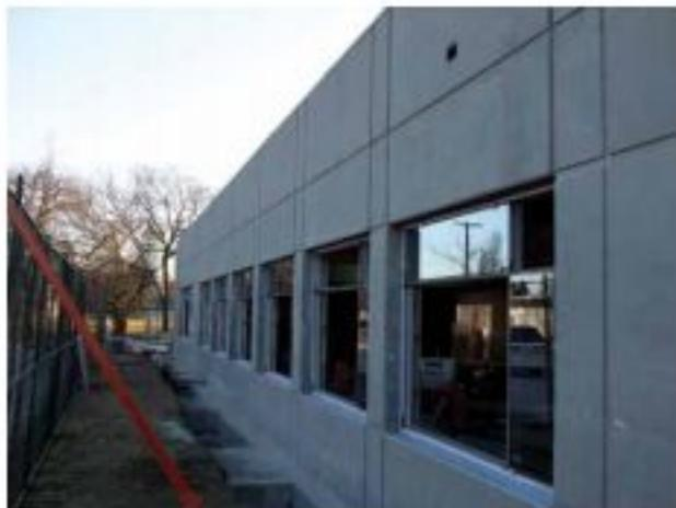
regardless of the extreme time constraints—due in part to a number of factors: cost, labor, and the challenges involved in effectively vibrating around numerous block-out recesses and reveals. Shotcrete proved to be not just the best solution, but the only solution! At the end of the day, the shotcrete process offered significant cost and time savings over conventional forming.
