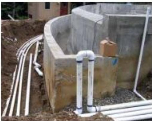
Large diameter plumbing to reduce water velocity and increase efficiency
