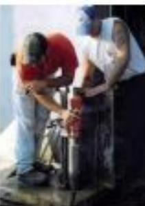
*The core drilling of a shotcrete panel to see the encapsulation of the reinforcing bars*
