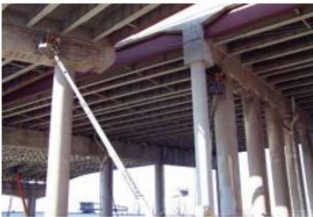
A 60 ft (18.28 m) boom lift was used to access piers
