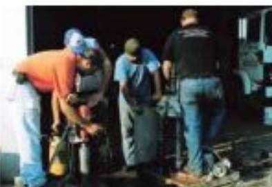
*The core drilling of the shotcrete panels to see the encapsulation of the reinforcing bar*
