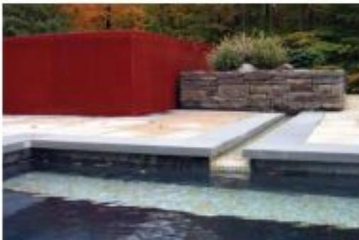
*Spa with red concrete panels overflowing to runoff into pool*
