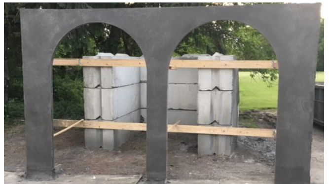
Fig. 3: Finished architectural shotcrete arch panels.
