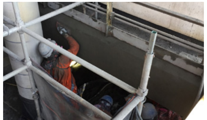
Fig. 8: Refinery crew cutting back freshly gunned shotcrete fireproofing
