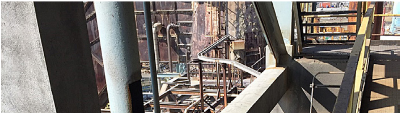
Fig. 4: Shotcrete fireproofing on beams and columns in FCCU.
