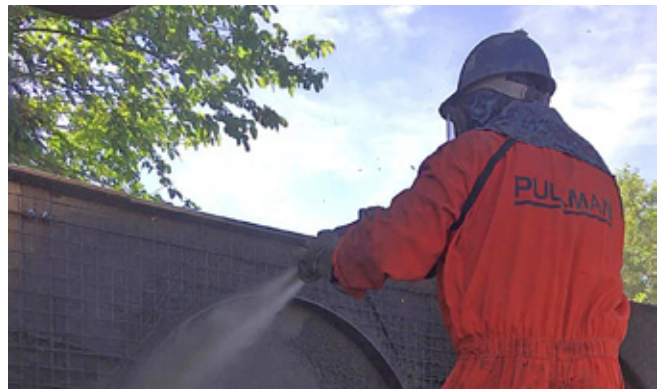
Fig. 2: Shotcrete application using dry-gun shotcrete process on architectural arch panels.
