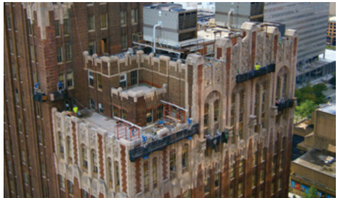
Fig. 7: Building envelope work on historical restoration project
