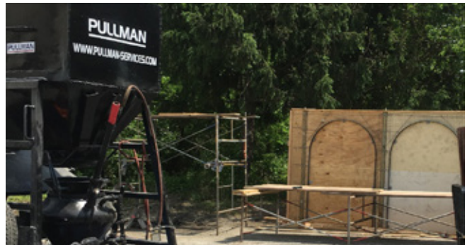
Fig. 1: Setup and form work for mock-up of an architectural shotcrete project.
