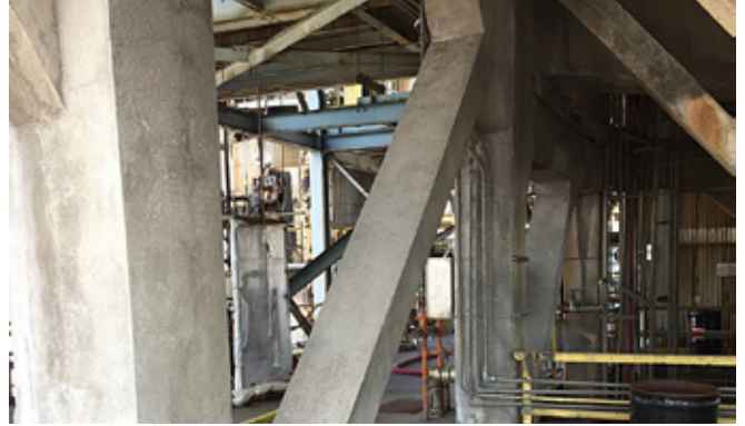
Fig. 5: Refinery fireproofing repairs
