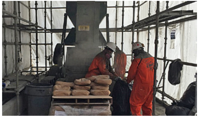
Fig. 6: Typical industrial shotcrete set-up for dry-mix process fireproofing
