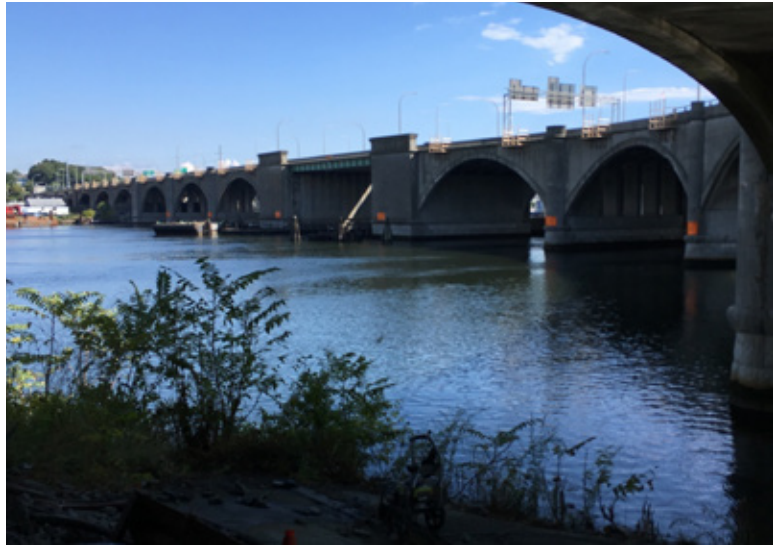
Fig. 5: Washington Bridge Concrete Repair
