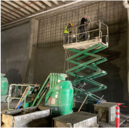
Fig. 4: Shear Wall Project
