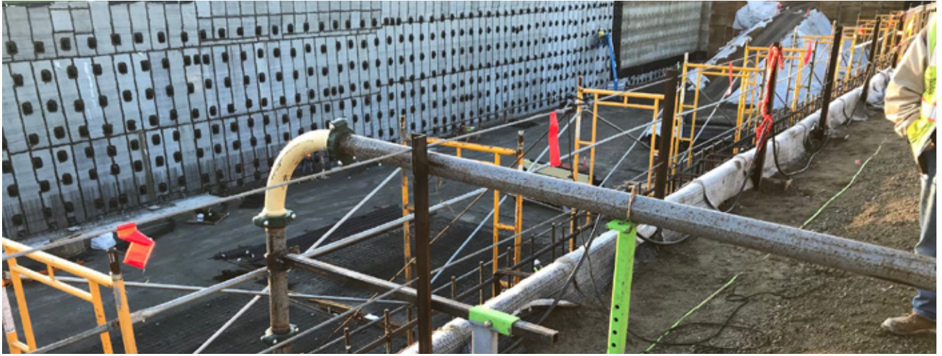
Fig. 3: Shotcrete standpipe clamp and support
