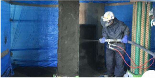
Fig. 3: Spraying of UHPFRC on air tubes
