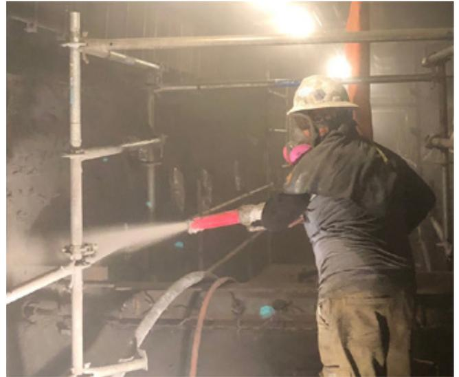
*Fig. 5: The respiratory protection worn during gunning operations fulfills the COVID-19 face mask directive.*
