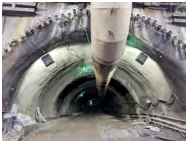
Fig. 2: Plymouth Tunnel East Portal top heading excavation
