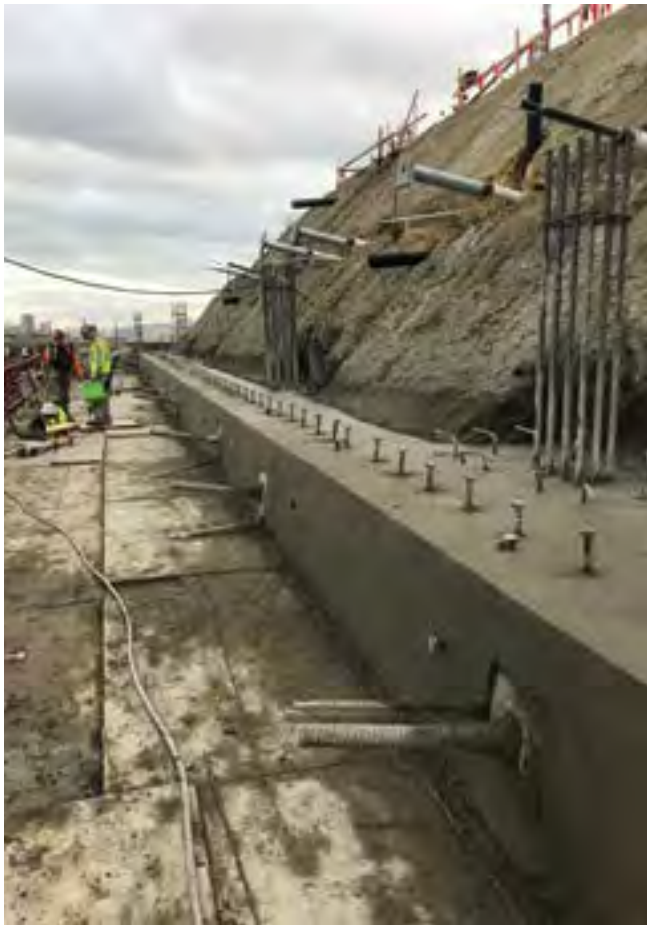
Fig. 3: Finishes on grade beam
