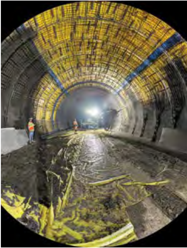
Fig. 9: Initial shotcrete application on PVC liner
