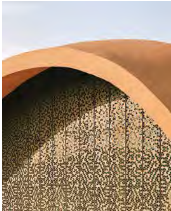
Fig. 3: Perforated corten screens, inspired by traditional Arabic mashrabiya, introduce filtered sunlight to the interiors (Photo courtesy of Rory Gardiner)
