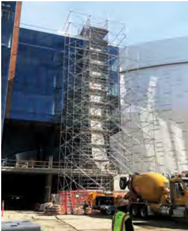
Fig. 3: Self-supporting scaffold tower
