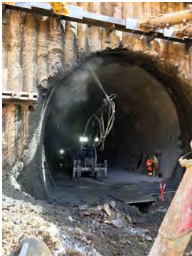
Fig. 4: Completion of initial lining after excavation
