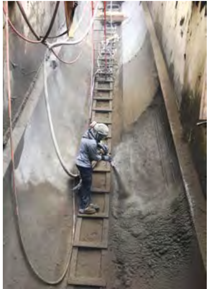
Fig. 4: Shooting side of basin off middle strip
