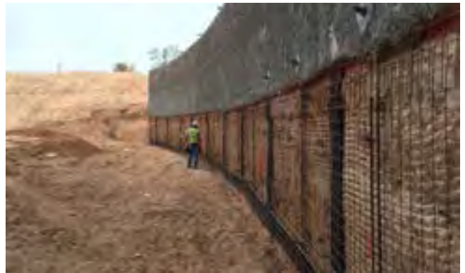
Fig. 3: Soil nail facing at Phoenix Children's Hospital on radius walls
