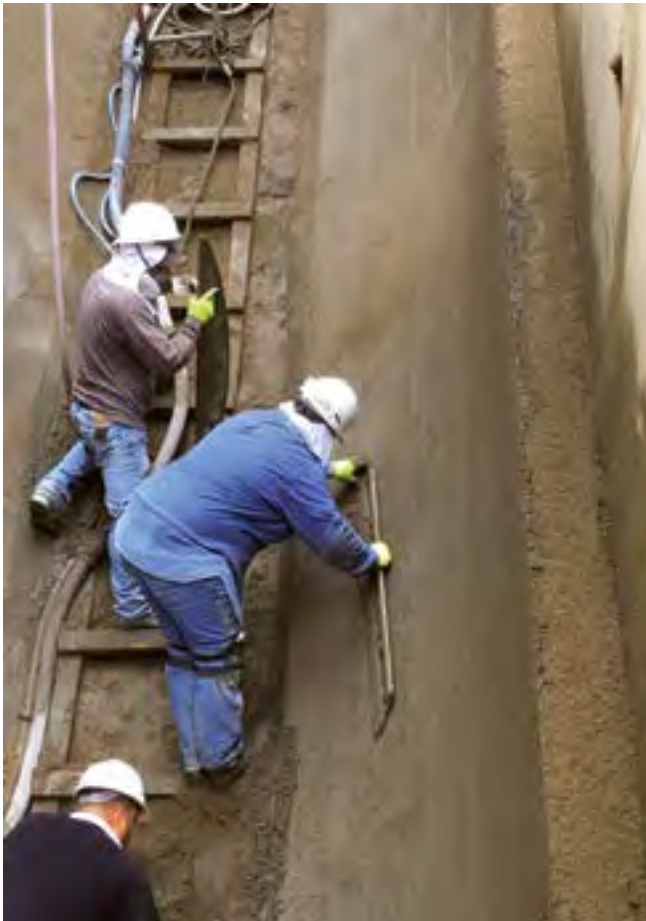
Fig. 3: Careful trimming of the sides
