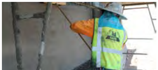
Fig. 7: Broom drag finish
