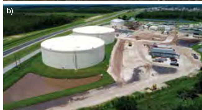
Fig. 3(a) and (b): CROM prestressed concrete tanks
