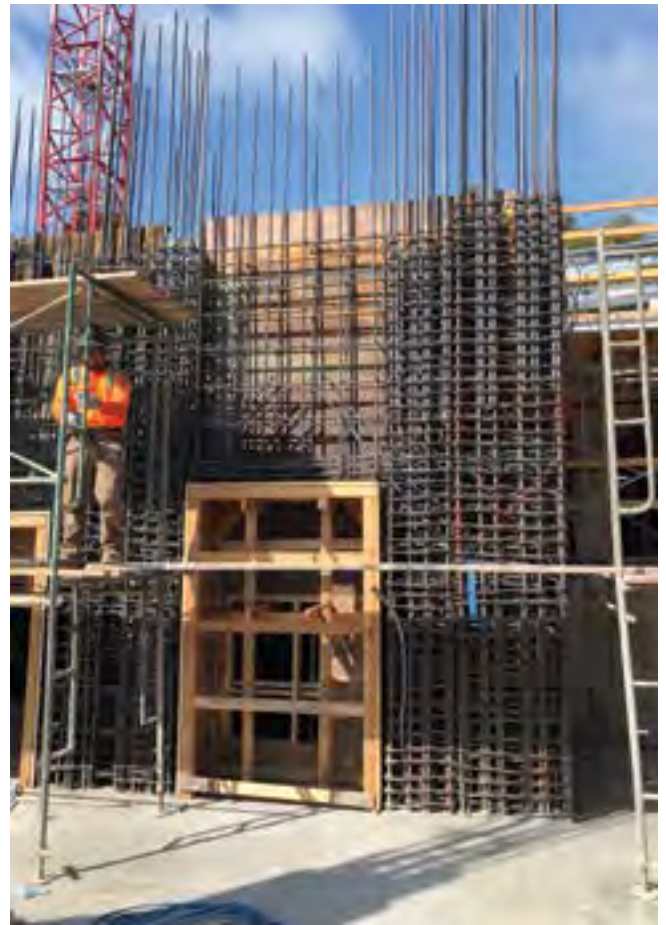
Fig. 4: Typical shear wall and boundary elements
