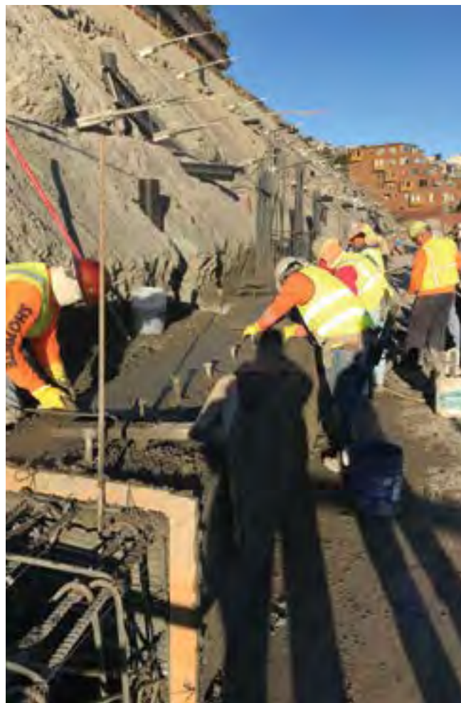
Fig. 2: Grade beam during shotcrete installation
