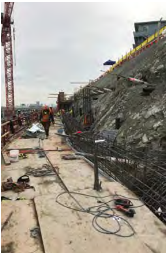
Fig. 1: Grade beam with work platform
