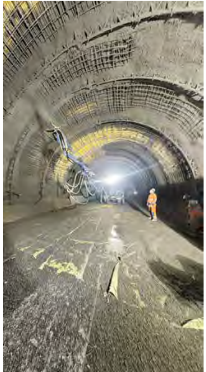
Fig. 7: Spraying secondary liner bays between arches
