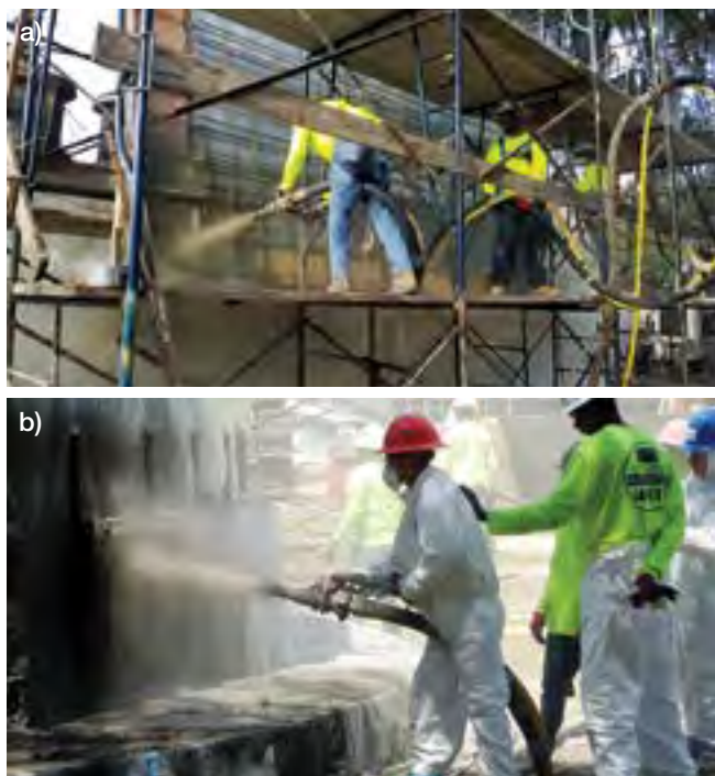
Fig. 4(a) and (b): CROM nozzlemen certification testing
