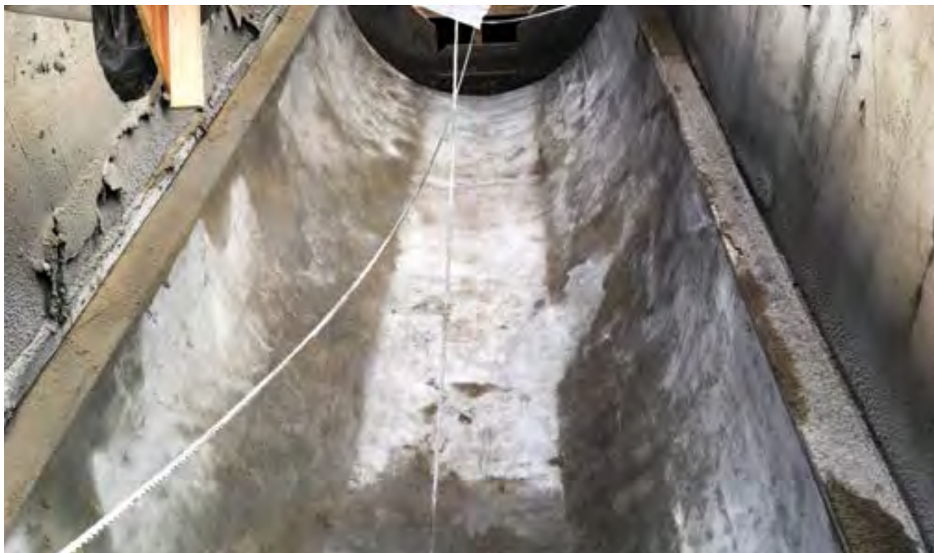
Fig. 1: Finished screw pump basin with tight radius
