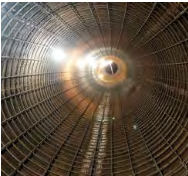
Fig. 4: Reinforcing bar installed
