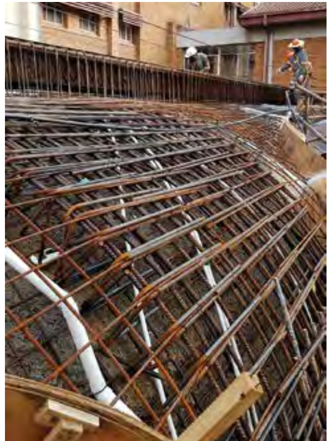
Fig. 3: Complex reinforcing steel for the canopy
