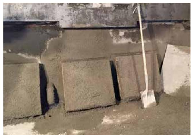
Fig. 2: Substrate panels after spraying
