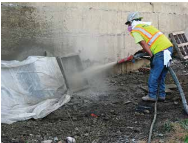
Fig. 1: Field test panel being properly gunned on site
