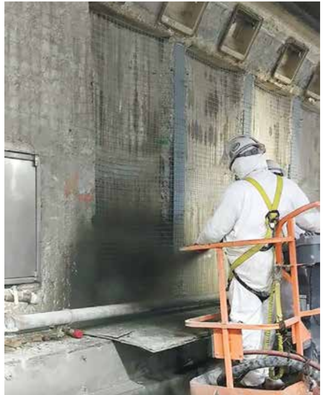
Fig. 3: During construction, repair of the drainage chases (Photo courtesy of Cruz)
