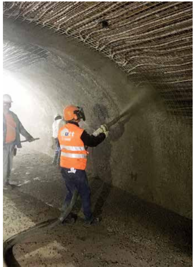
Fig. 2: MAPEI's UTT products have commercial as well as industrial applications. Its additive technology was added to shotcrete to create the walls of this high-tech wine cave
