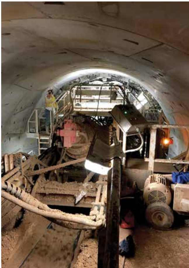
Fig. 1: MAPEI's UTT products were used to help a tunnel boring machine dig the Anacostia River Tunnel, which extends for 2.37 miles (3.81 km) from Robert F. Kennedy Stadium in northeast Washington, DC, to Poplar Point in southeast DC
