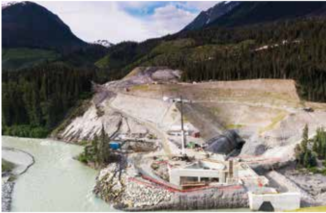
Fig. 1: Upstream tunnel portal for Upper Lillooet Hydroelectric project
