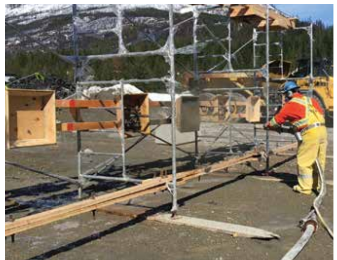
Fig. 7: Hand-nozzling qualification for dry-mix shotcrete
