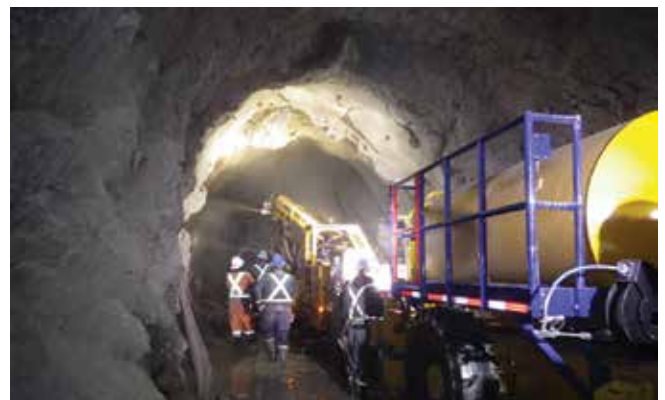
Fig. 6: Robotic sprayer applied wet-mix shotcrete at the tunnel heading
