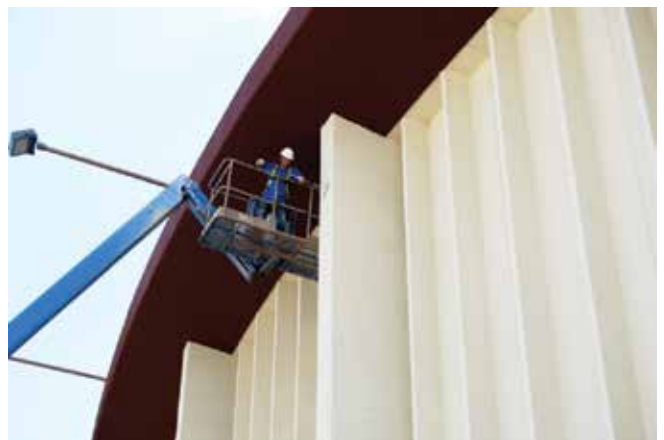
Fig. 4: Applying elastomeric coating to concrete ring beam
