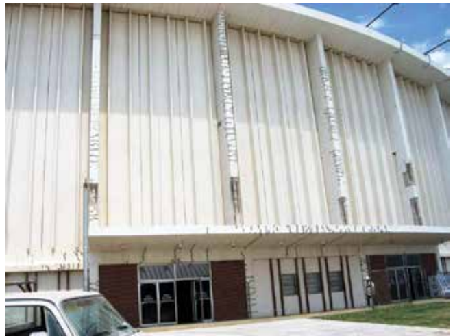
Fig. 3: Epoxy injection and removal of delaminated concrete of concrete columns
