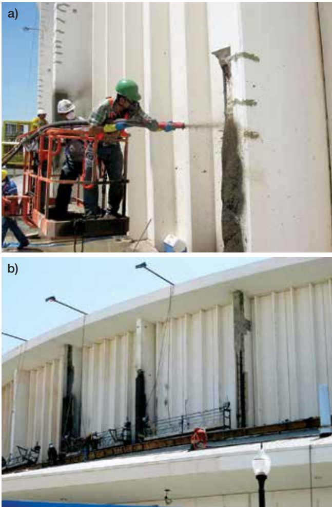
Fig. 7(a) and (b): Dry-mix shotcrete installation
