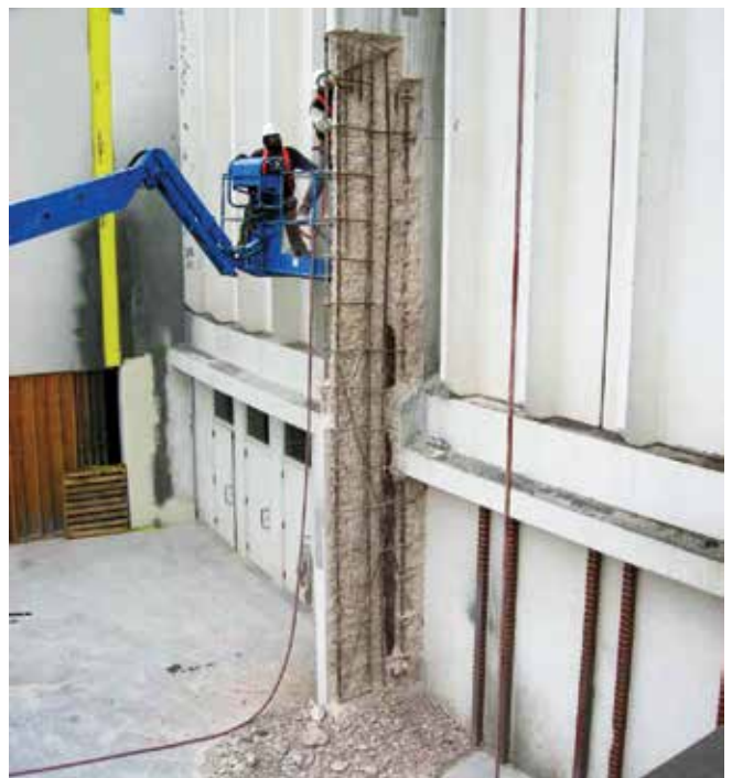
Fig. 5: Demolition of delaminated concrete
