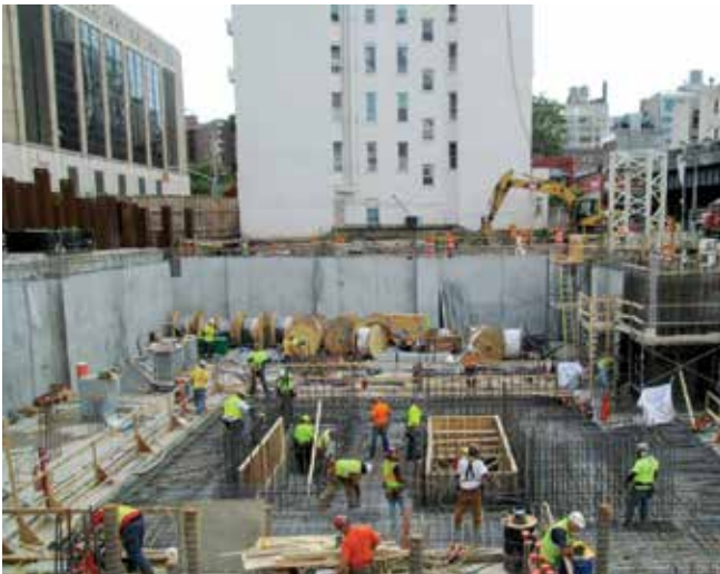
Fig. 1: Hudson Yards, 12,000 lb/in. 2 (83 MPa) foundation
