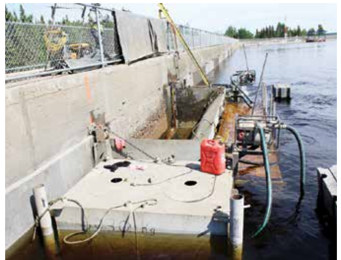
Fig. 2: Mobile cofferdam system on dam repair project
