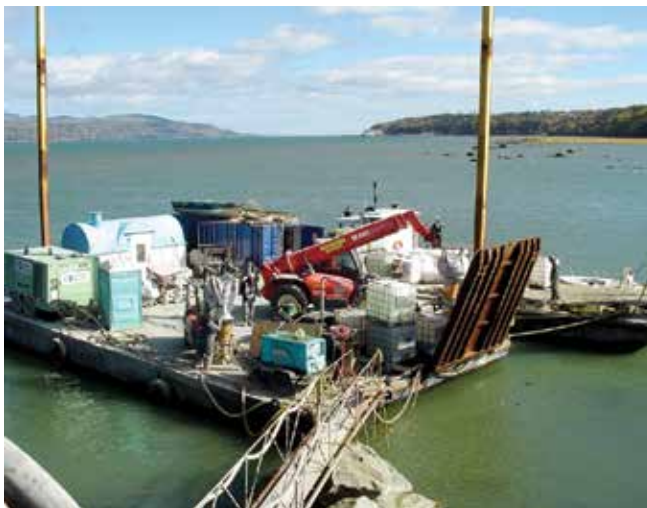
Fig. 1: Shotcrete material and equipment transported by barge
