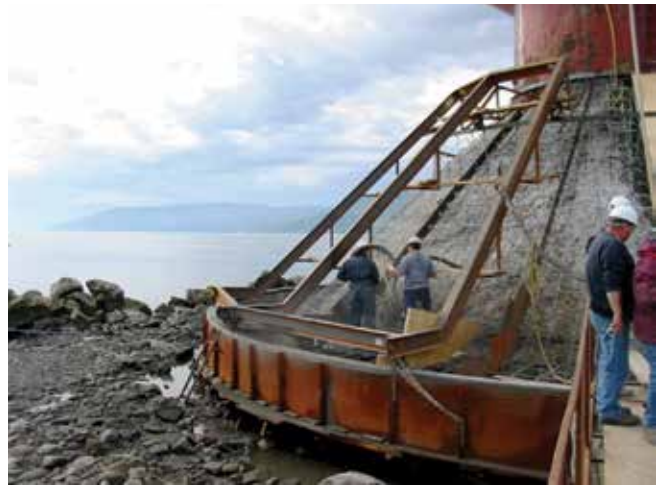
Fig. 4: Lighthouse foundation repair with abrasion-resistant shotcrete
