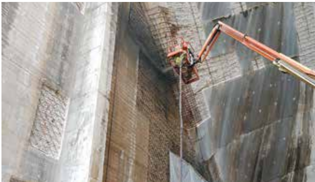
Fig. 4: Dry-mix shotcrete and water hose secured to the manlift basket 60 ft (18 m) in the air (Buchanan Dam, Llano County, TX)
