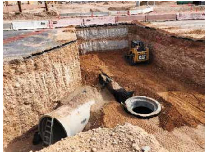
Fig. 11: Backfilling of the culvert
