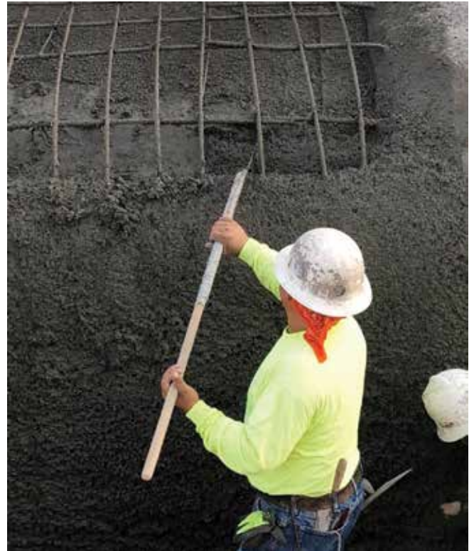
Fig. 6: Cleaning and roughening the construction joint before shotcrete placement starts on the top of the arch
