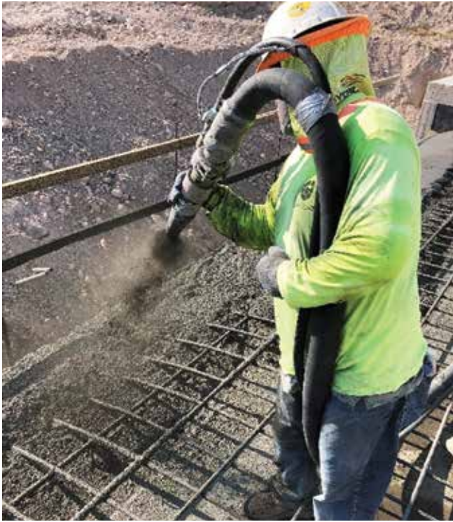
Fig. 7: Shooting the top section of the arch
