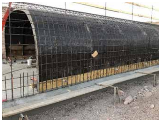
Fig. 3: Reinforcing steel in place over the supporting arch form
