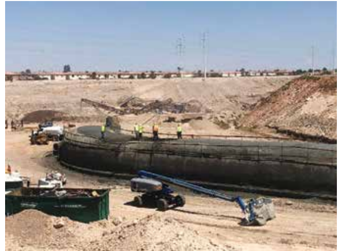
Fig. 8: An overview of shooting the top of the arched culvert
