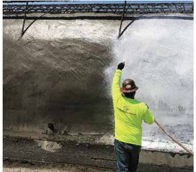
Fig. 10: A membrane curing compound being sprayed on the fresh shotcrete surface
