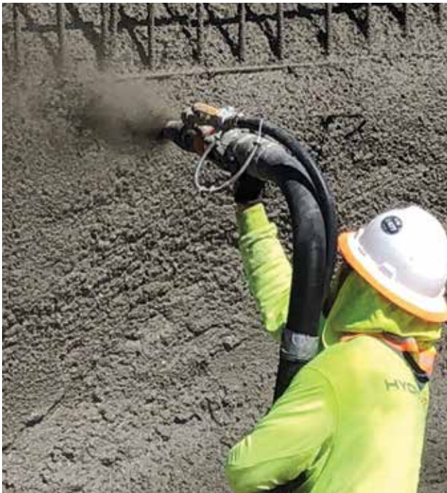
Fig. 5: Shotcrete placement further up the arched wall
