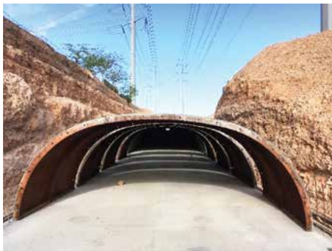
Fig. 2: Forms ready to receive reinforcing steel
