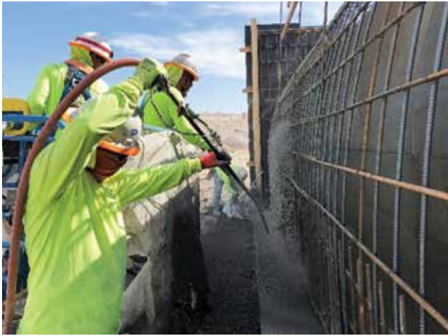
Fig. 4: Shotcrete placement starting at the bottom of the arched wall
