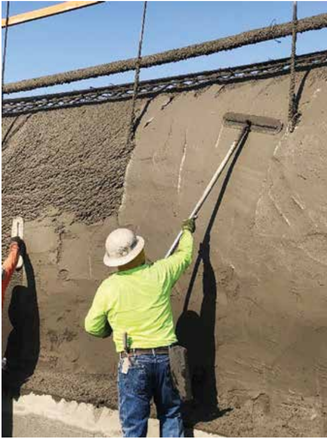
Fig. 9: A fresno trowel finish is provided on the shotcrete surface
