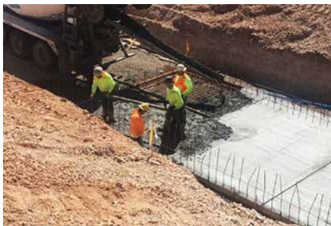
Fig. 1: Casting the arched culvert floor
