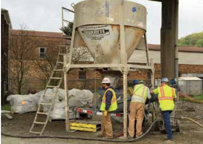
Fig. 6: Equipment setup for gunning prepackaged material
