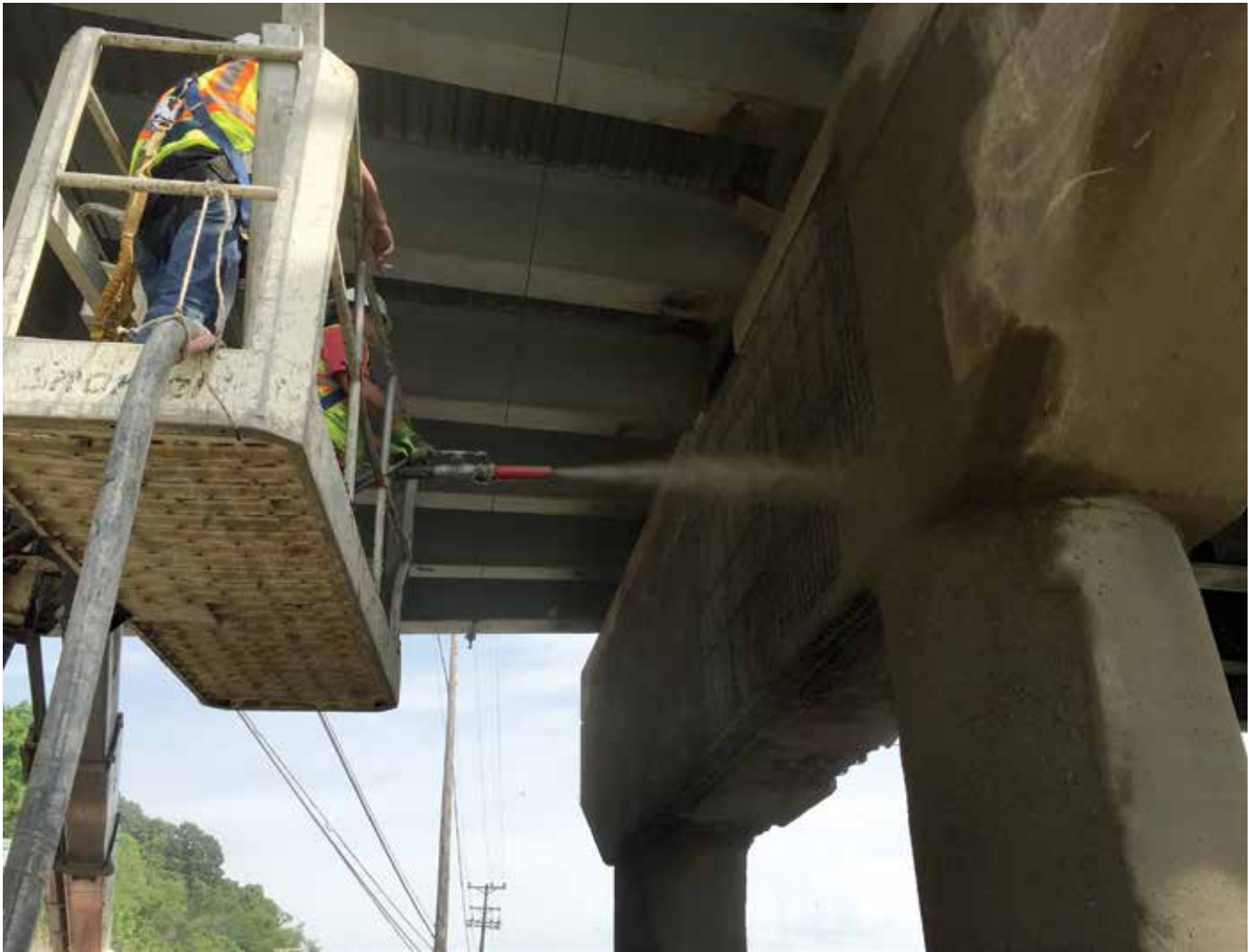
Fig. 4: Dry-process shotcrete placement on a bridge pier
