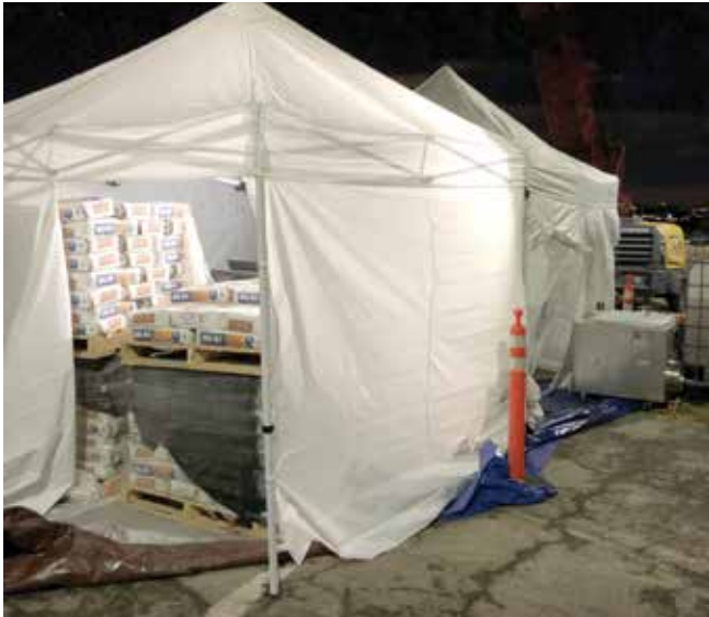
Fig. 6: A part of Eastco's laydown on the apron of Pier 40
