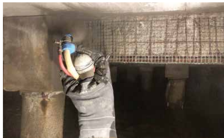
Fig. 3: An ACI Certified Nozzleman applying shotcrete to a Type 3 repair
