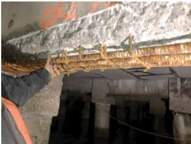
Fig. 1: A Type 3 repair after deteriorated concrete was removed
