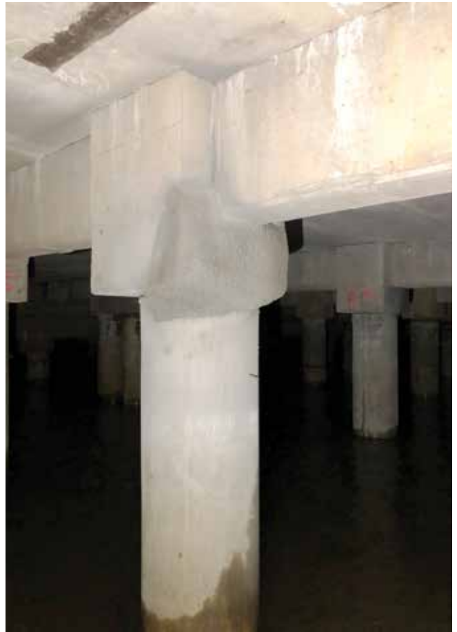
Fig. 4: A completed Type 4 repair
