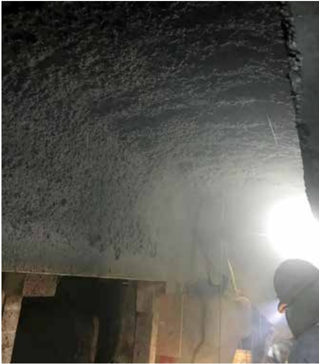
Fig. 3: Shotcreting in limited space under pier
