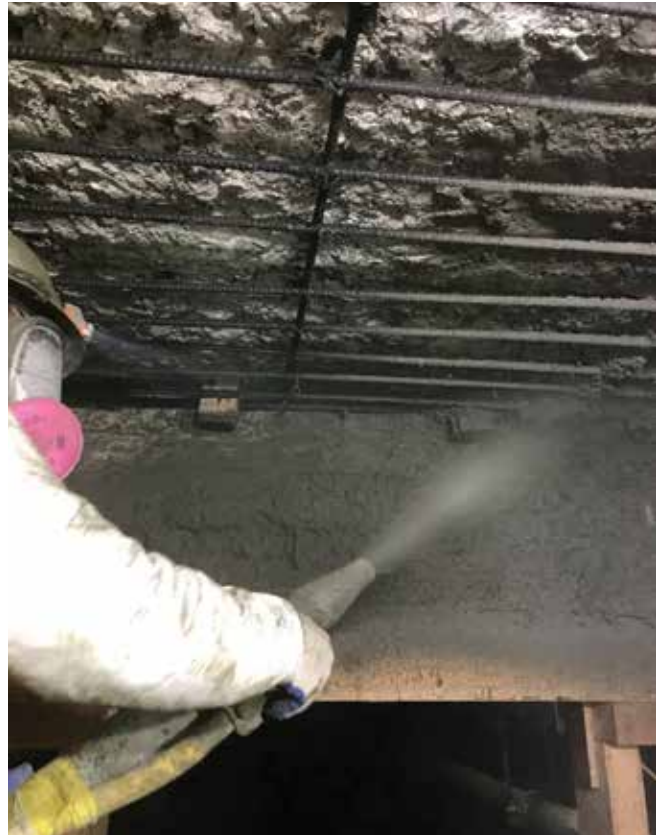
Fig. 4: Shooting on underside of pier
