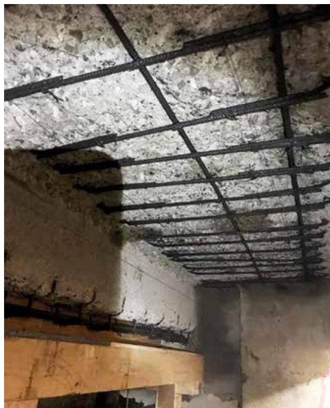
Fig. 2: Underside of pier ready for shotcrete
