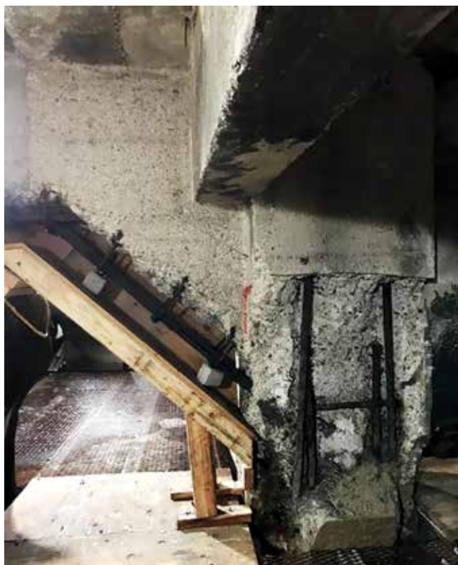
Fig. 1: Beam side prepared for shotcreting with minimal formwork
