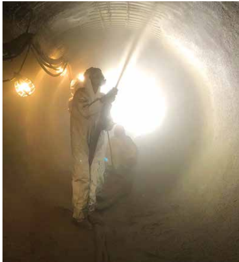
Fig. 5: Dry-mix shotcrete application in hydro penstock
