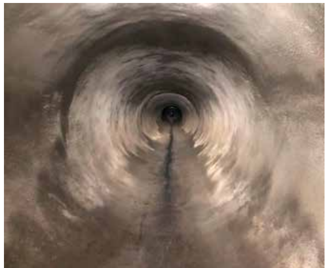
Fig. 4: Finished penstock shotcrete
