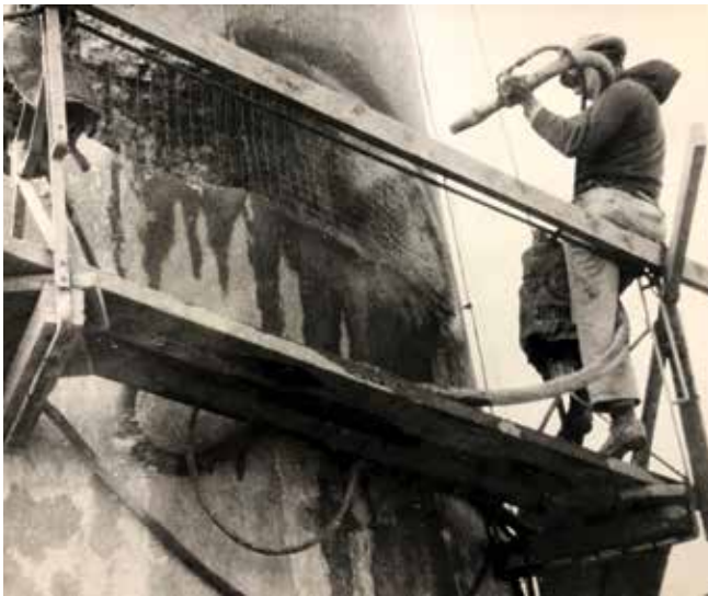
Fig. 1: Dry-mix shotcrete repair on a paper mill stack (image from 1960s)
