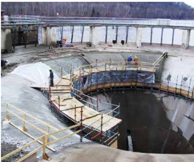
Fig. 2: Scaffolding for Glory Hole Spillway
