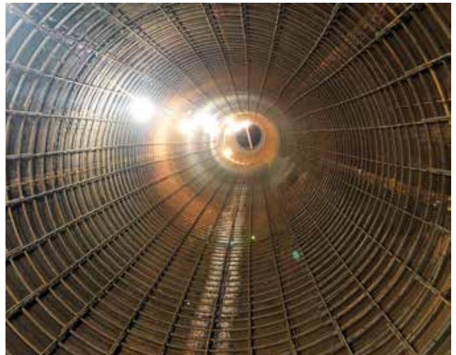
Fig. 3: In-house engineered structural reinforcement bar for a penstock shotcrete liner
