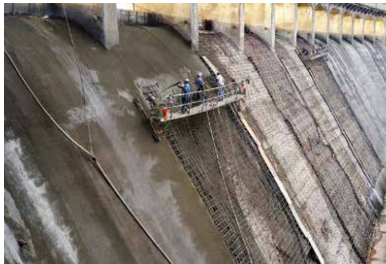
Fig. 6: Stevenson Dam Spillway resurfacing
