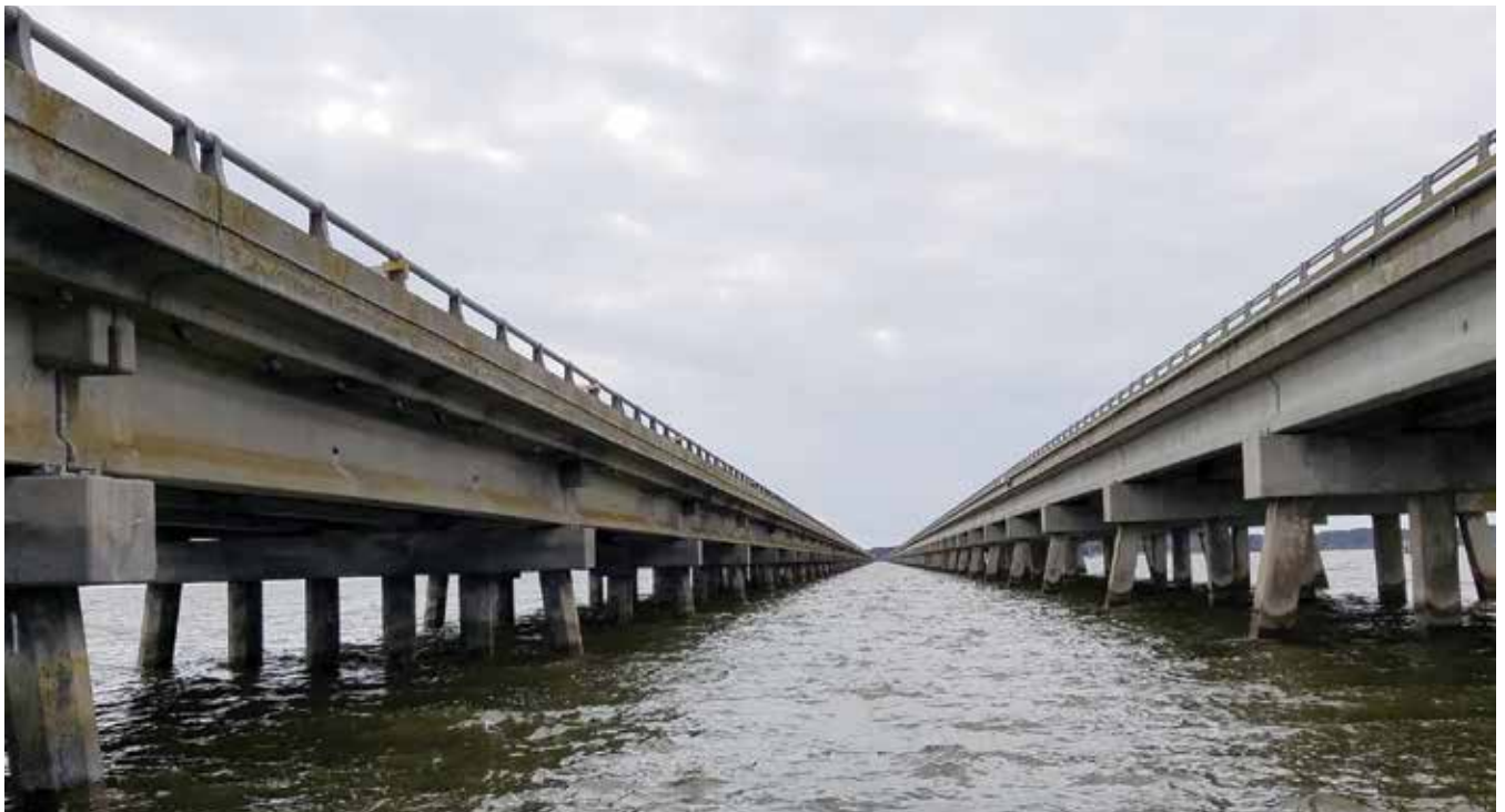
Fig. 1: The Wright Memorial Bridge
