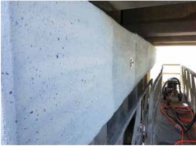
Fig. 6: Finished application of zinc anode and testing plate
