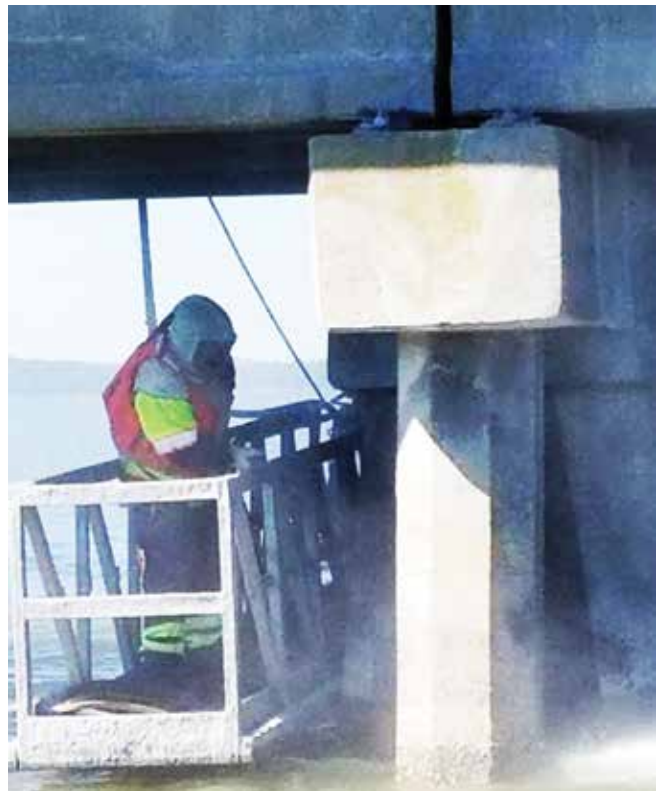
Fig. 5: Preparing to apply zinc anode
