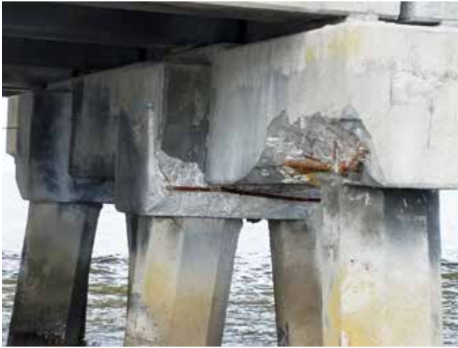
Fig. 2: Repair location on bent cap
