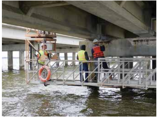
Fig. 4: Coastal Gunite Construction Company and Inspector testing for continuity
