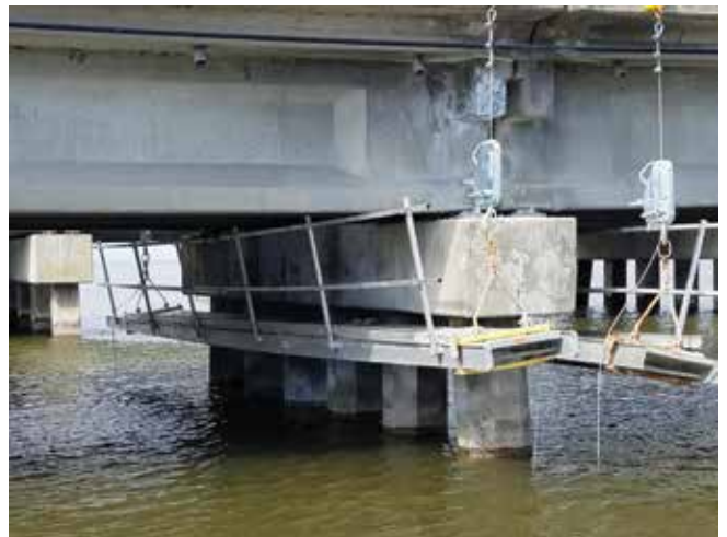
Fig. 9: Swing stage scaffolding
