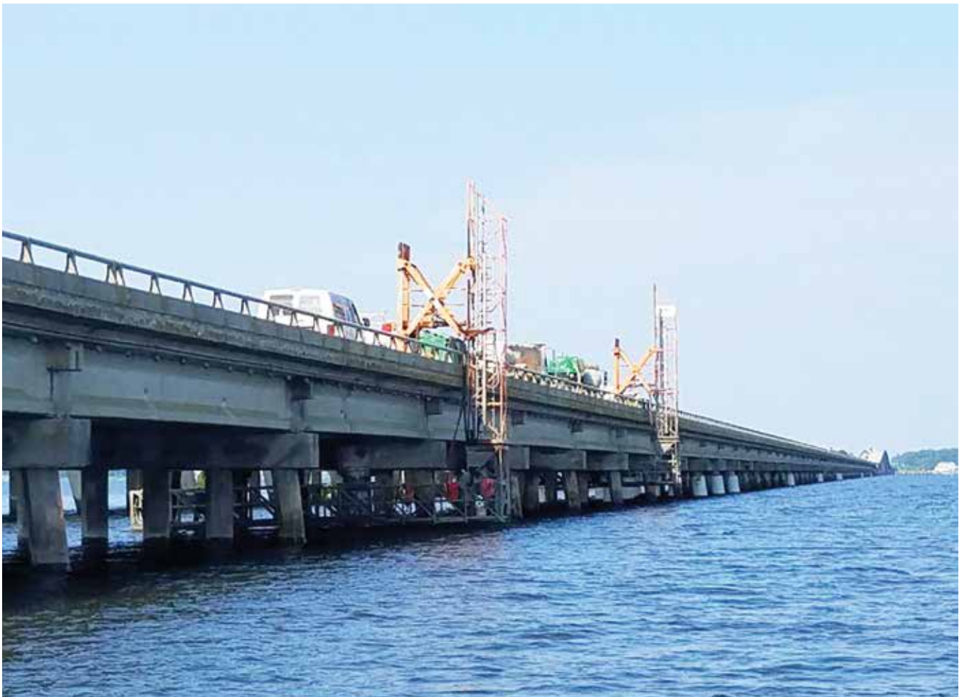
Fig. 7: Anderson Hydra-Platform Bridge Access Machines in use
