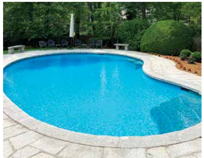
Fig. 5: Finished pool after renovation
