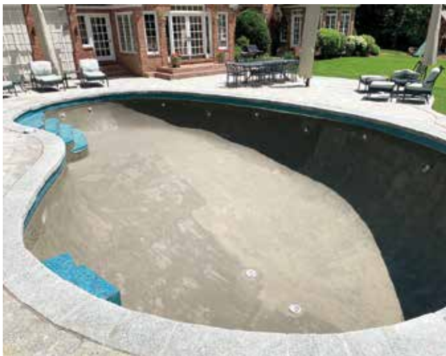
Fig. 4: Installation of waterproofing coat
