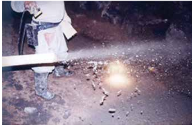
Fig. 4: Shotcrete is pneumatically projected concrete accelerated to high speed before impact on the receiving surface
