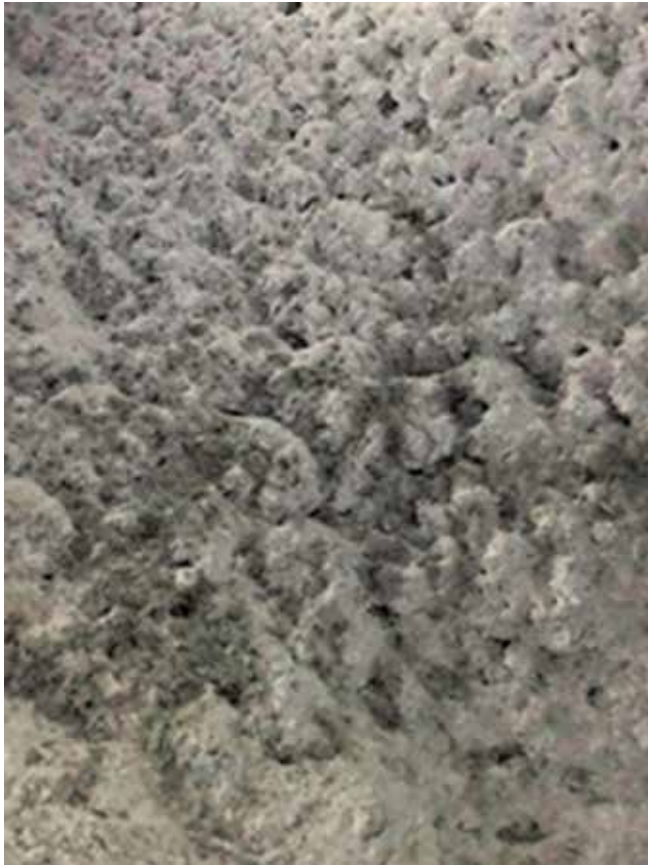
Fig. 3: Proper surface preparation is vital for successful application of shotcrete
