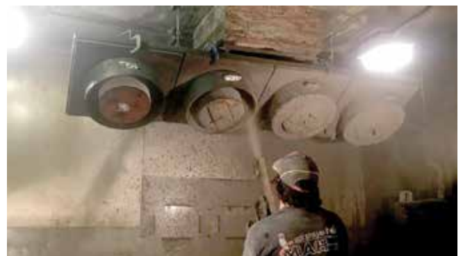
Fig. 6: Shotcrete being sprayed into inclined AASHTO T 344 rings
