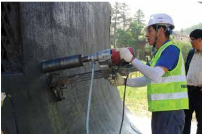
Fig. 8: Diamond drilling extraction of first core
