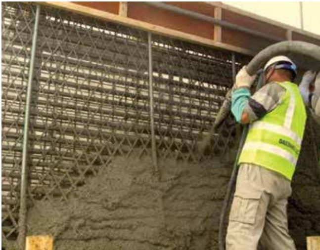
Fig. 4: Shotcrete applied to the coved area of the high wall
