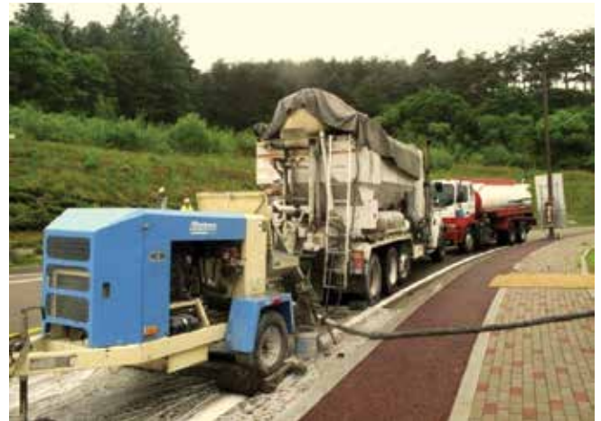
Fig. 3: Bench gun shooting shotcrete in high wall
