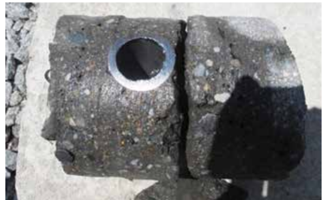
Fig. 17: Side view of core No. 7 from high wall cove. Shotcrete typically well consolidated and assigned ACI Core Grade No. 2
