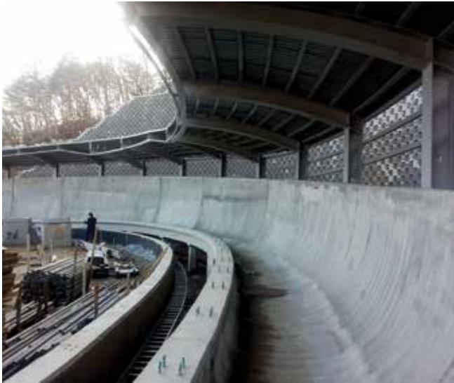
Fig. 18: Sliding track under construction
