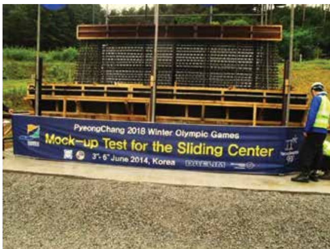
Fig. 1: General view of track mockup prior to shotcrete construction
