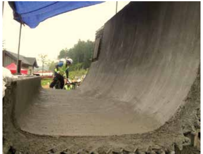
Fig. 6: Completed mockup after application of broom finish texture
