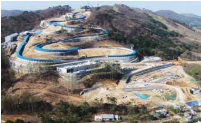
Fig. 19: Overview of completed sliding track
