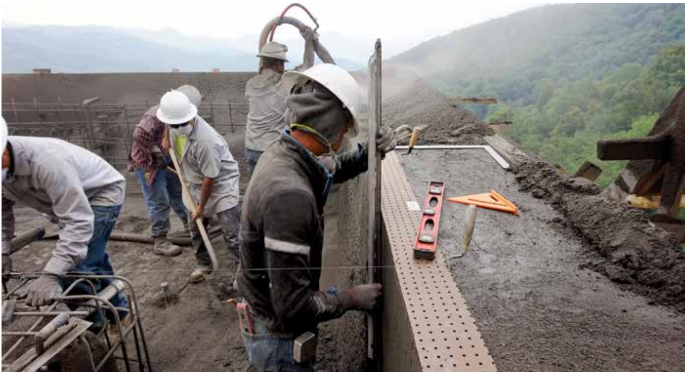
Example of dry-mix crew working safely in an active environment | Crew: Revolution Gunite | Photo: Ryan Oakes
