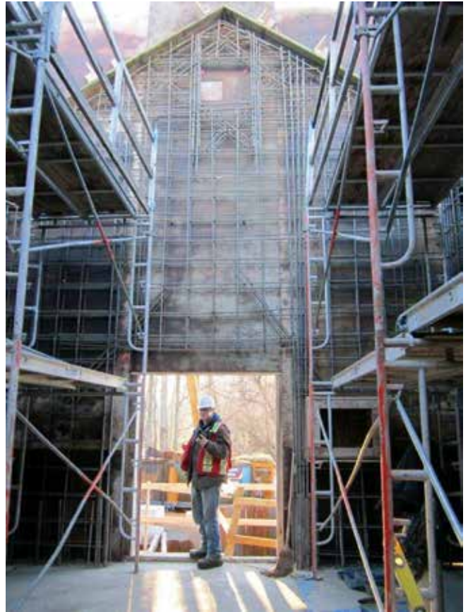
Properly installed reinforcing bar, formwork, and waterproofing
