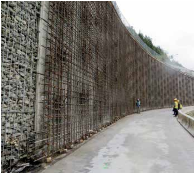
Properly installed reinforcing bar, formwork, and waterproofing
