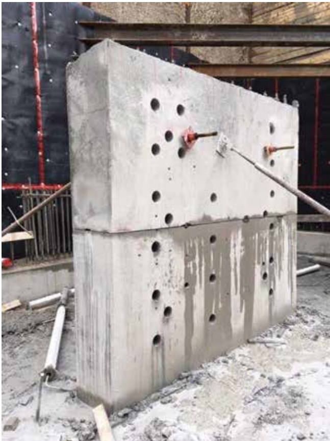
Structural shotcrete mockup
