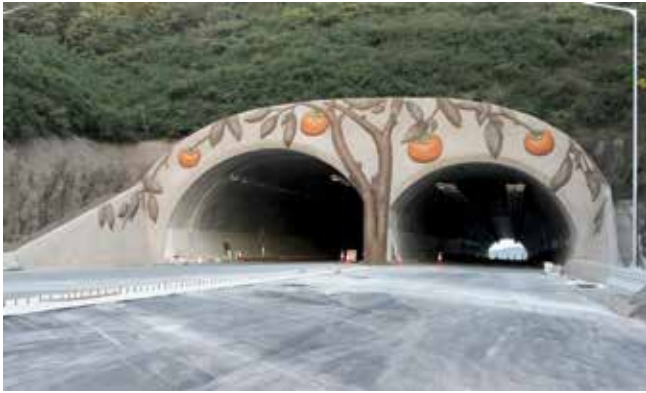
Fig. 5: Regionally symbolic tunnel portal built with cellular sprayed concrete
