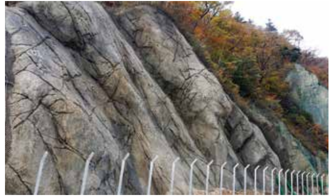
Fig. 6: Artificial rock slope stabilization with cellular sprayed concrete
