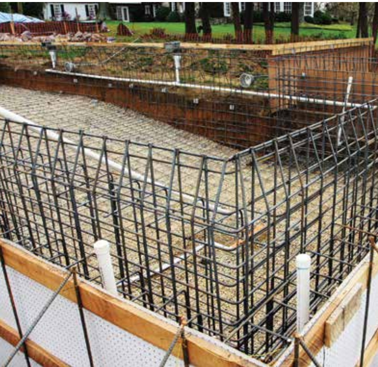
Fig. 5: An example of good reinforcing bar placement
