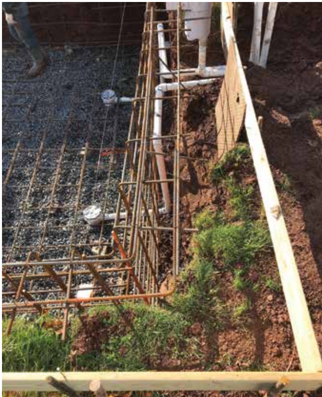
Fig. 1: Not enough reinforcing bars, and improper layout
