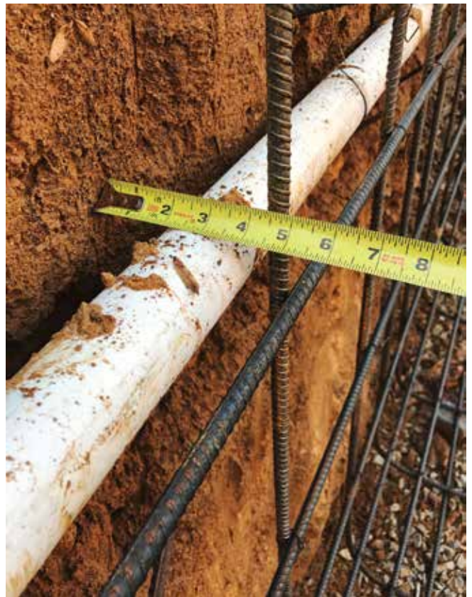
Fig. 3: Not enough cover over the reinforcing bars
