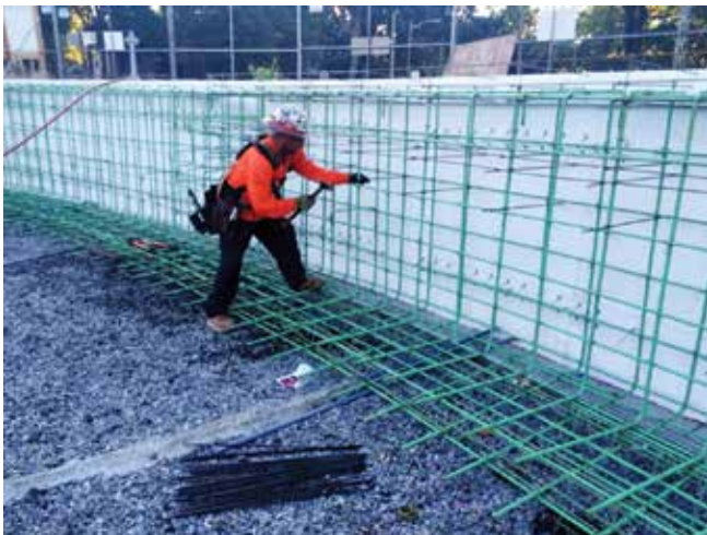
Fig. 1: Setting pencil rod for grade control
