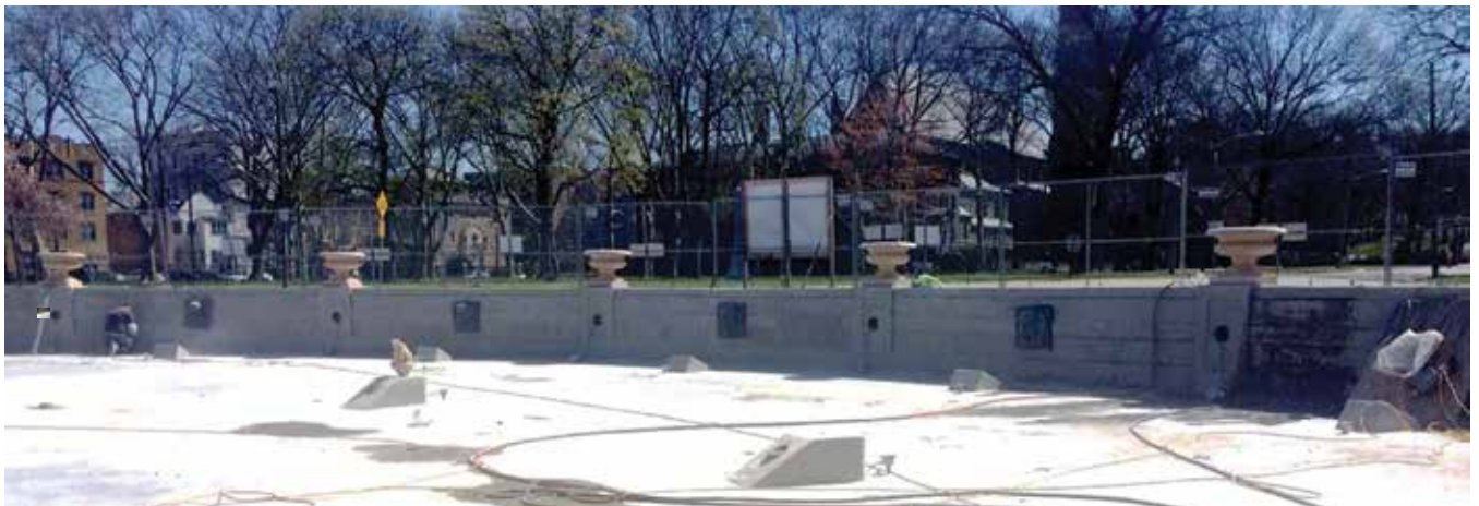
Fig. 5: East quadrant completed
