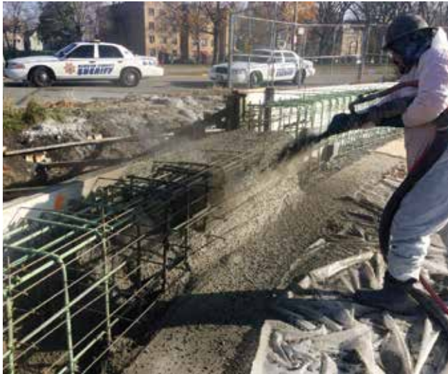
Fig. 4: Shotcrete placement in outer basin wall
