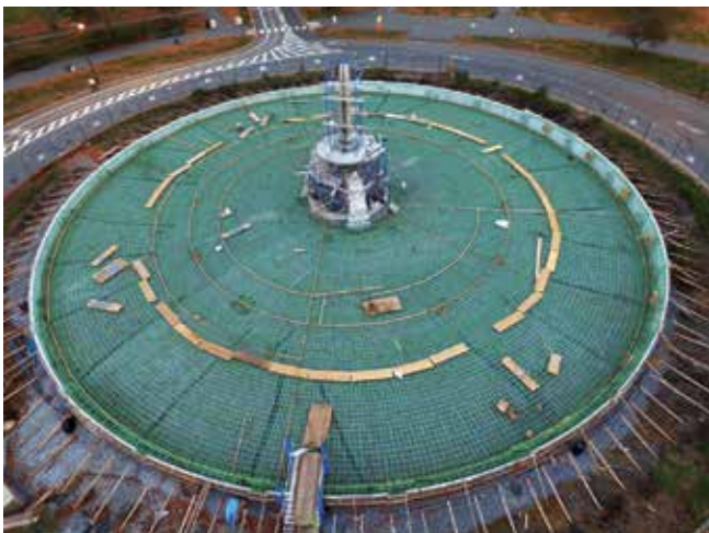
Fig. 2: Overview before concrete placement
