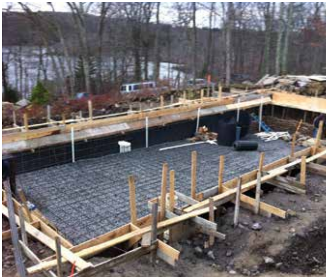
Fig. 2: Lightweight, one-sided form is all that is needed when using shotcrete
