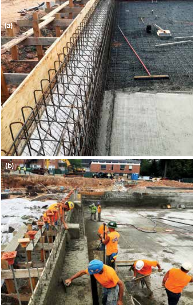
Fig. 4(a) and (b): Shotcrete on top of cast floor
