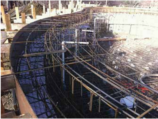
Fig. 5: Lightweight curved form with steel reinforcing for radius steps
