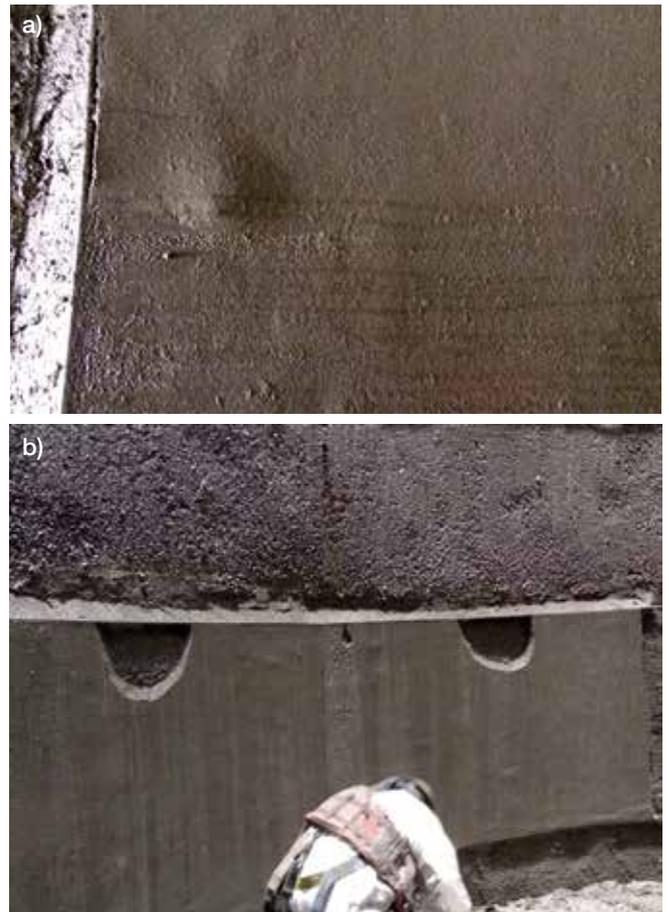
Fig. 18: (a) Water pressure buildup at the back of the finish course shotcrete; and (b) the shotcrete popouts were cut off and repaired with shotcrete when the shaft was dry
