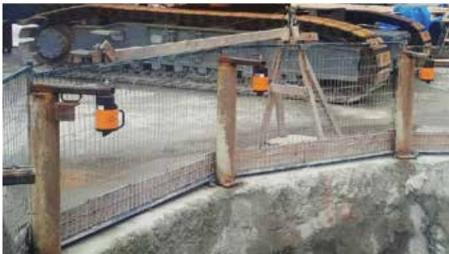
Fig. 4: North shaft slurry wall with steel columns and laser setup
