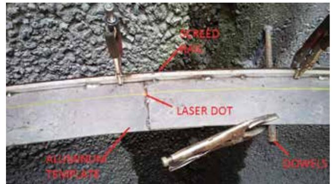
Fig. 6: Screed rail installation (looking down)
