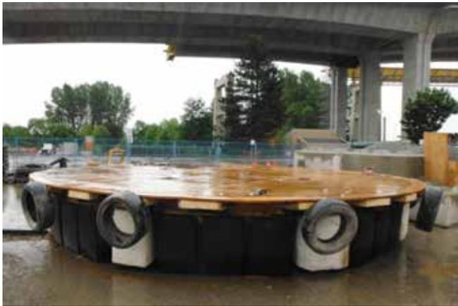
Fig. 8: Floating platform during shotcrete application
