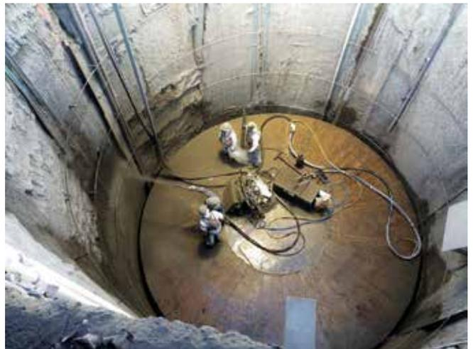
Fig. 16: Birds-eye view of dry-mix shotcrete application from the floating deck. Note the low dust and simple setup of the shotcrete operation. Horizontal screed rails to control the base course thickness were spaced at 1.5 m
