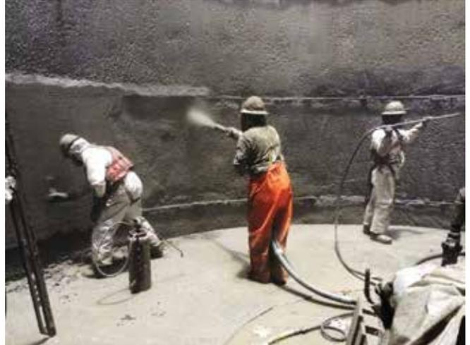
Fig. 15: Application of finish coat dry-mix shotcrete from floating deck
