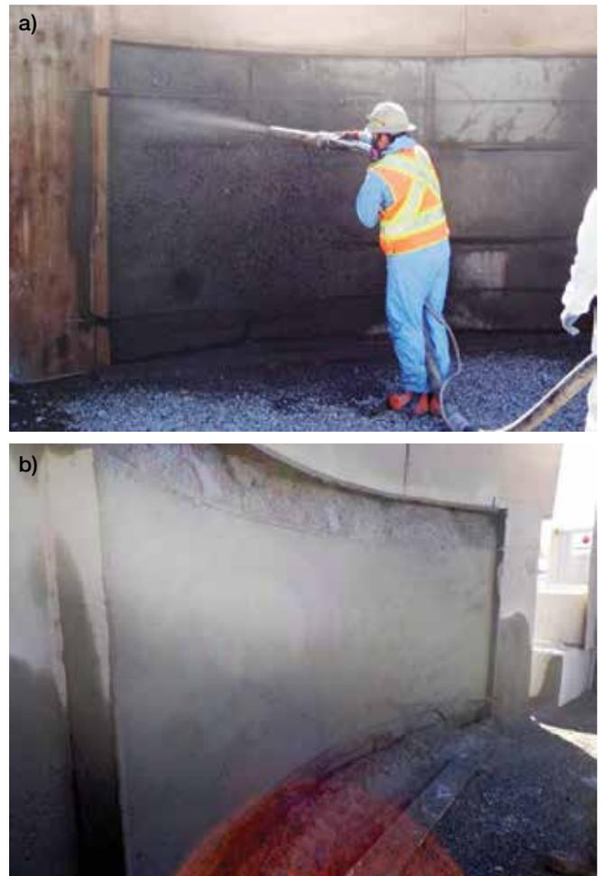
Fig. 10: Preconstruction mockup panel: (a) shooting mockup panel; and (b) closer view of mockup panel
