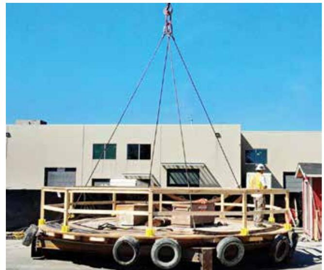
Fig. 7: Crane-lifted platform during rail installation
