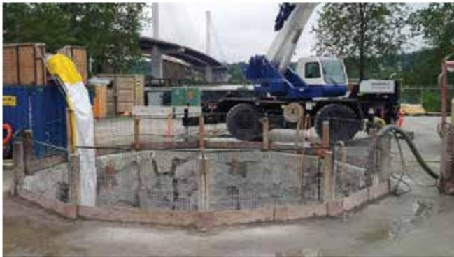
Fig. 3: North shaft slurry wall—Coquitlam, BC, Canada
