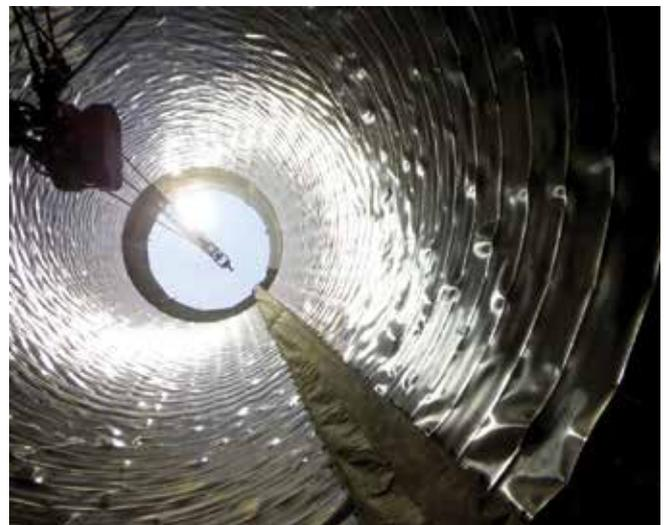
Fig. 2: Completed shotcrete wall with plastic slip liner installed
