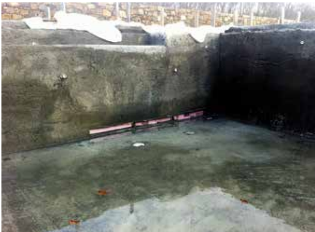
Fig. 4: Formed toe-kick recesses for the pool and spa circulation systems
