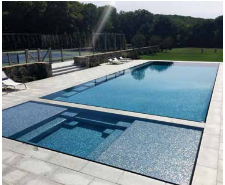
Fig. 6: Completed pool and spa
