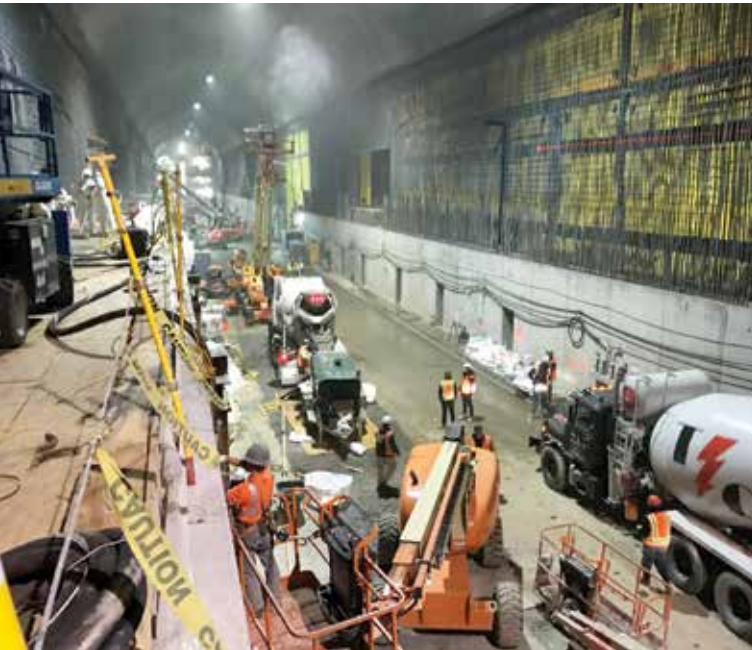
Fig. 14: CM007 Cavern walls; this is one of two caverns
