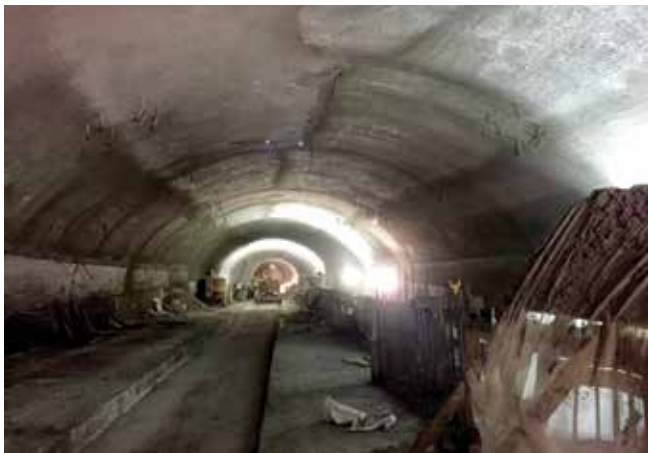
Fig. 7: Rod-finished cavern at CM006
