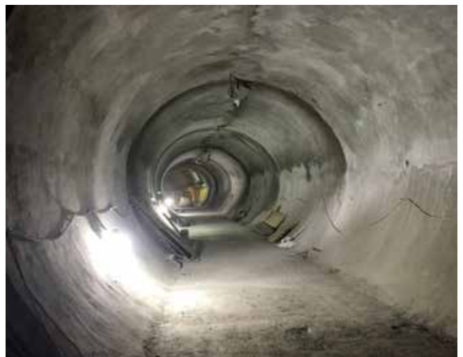
Fig. 11: Completed CM005 tunnel section
