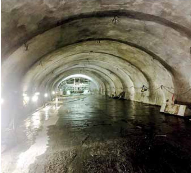
Fig. 12: Finished Access Tunnel 1 with rubber float finish
