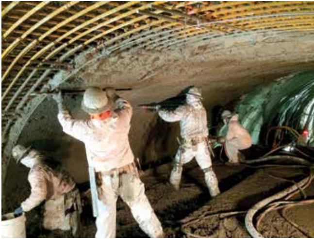
Fig. 3: Finishing at CQ39, cutting out pencil rod and starting to float
