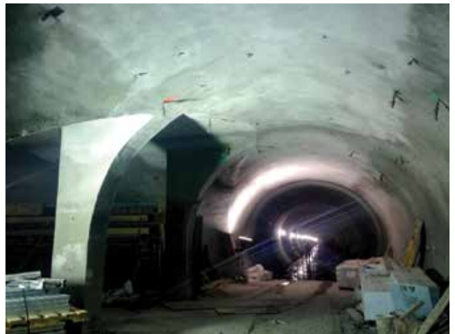
Fig. 10: Upper level arch of TT#1 structure, tunnel, and cross passage interface
