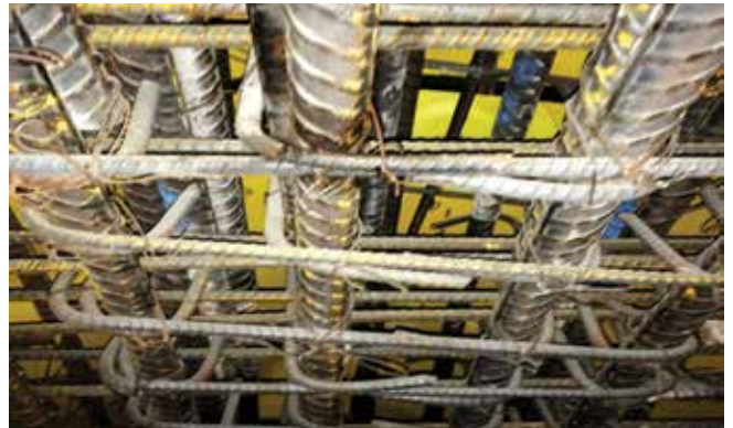
Fig. 9: Reinforced beam section in upper level arch of CM005 TT#1 structure
