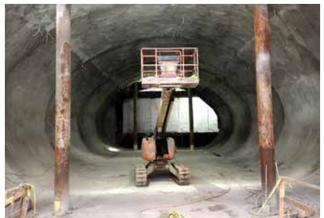
Fig. 2: CQ39 Tunnel section, prior to cutting out support columns
