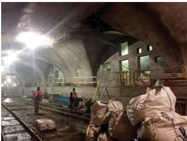
Fig. 8: Communications room with fishmouth, interior wall, and arched ceiling at CM006
