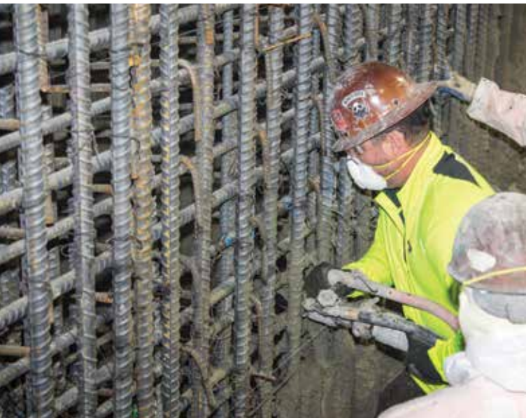
Fig. 15: CM007 Cavern walls; 3.5 ft (1.1 m) being placed
