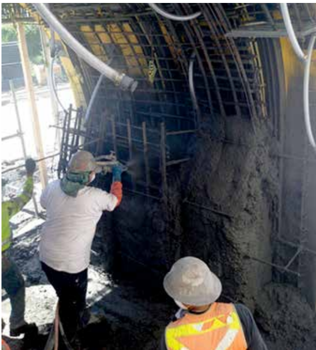
Fig. 6: Preconstruction field trial PAC mockup and hand spraying of vertical walls
