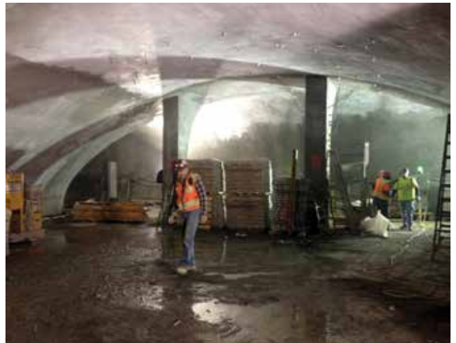
Fig. 3: Typical example of PAC lined structure
