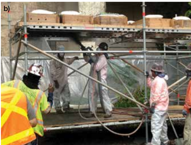
Fig. 5: Preconstruction test panels: (a) vertical; and (b) overhead
