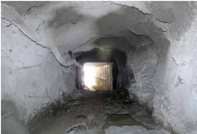
Fig. 7: Final layer of permanent shotcrete in place
