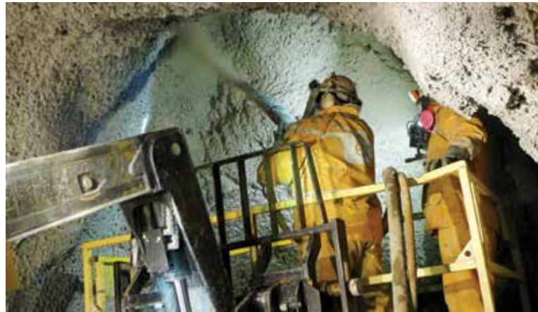
Fig. 5: Shotcrete placement in high back
