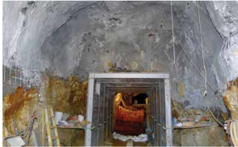
Fig. 4: Installing steel sets under initial shotcrete support
