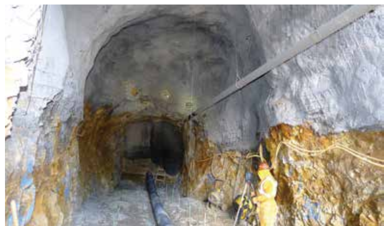
Fig. 2: Portal area excavated and initial support in place
