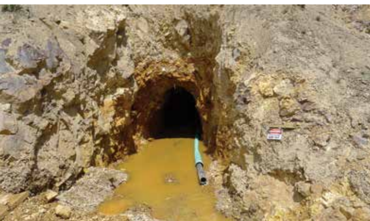
Fig. 1: Portal before rehabilitation
