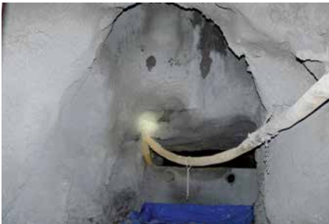
Fig. 8: Final shotcrete in place at high back
