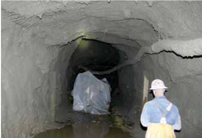
Fig. 6: Initial layer of permanent shotcrete support
