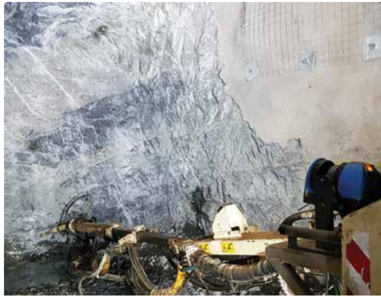
Fig. 1: Monitoring equipment on a shotcrete rig
