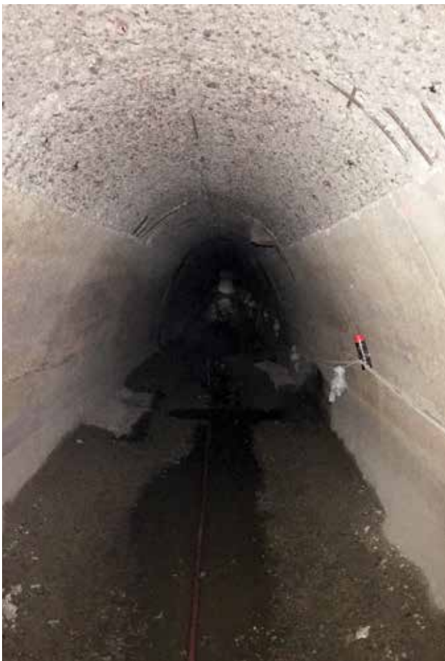
Fig. 3: Tunnel after hydrodemolition
