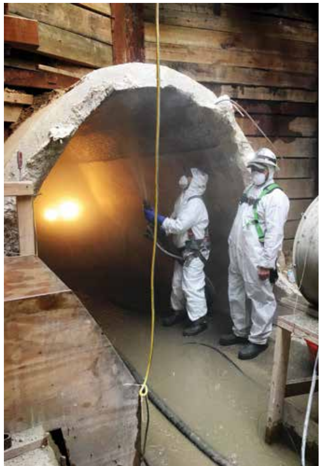
Fig. 4: Tunnel being shotcreted after surface preparation
