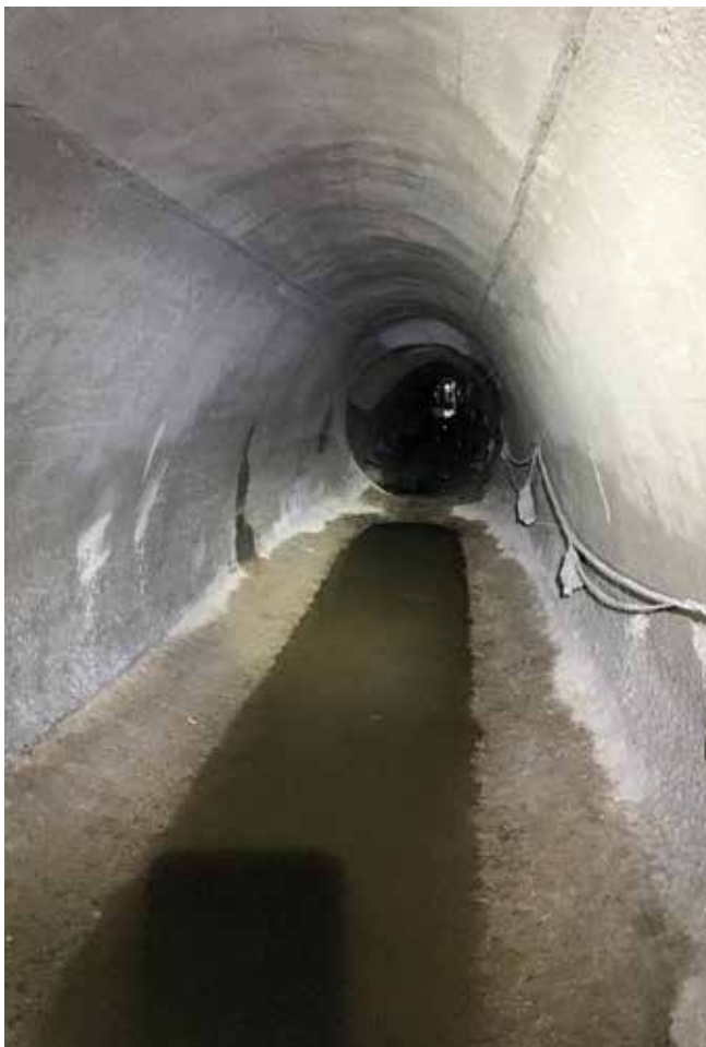
Fig. 1: Finished tunnel crown installation
