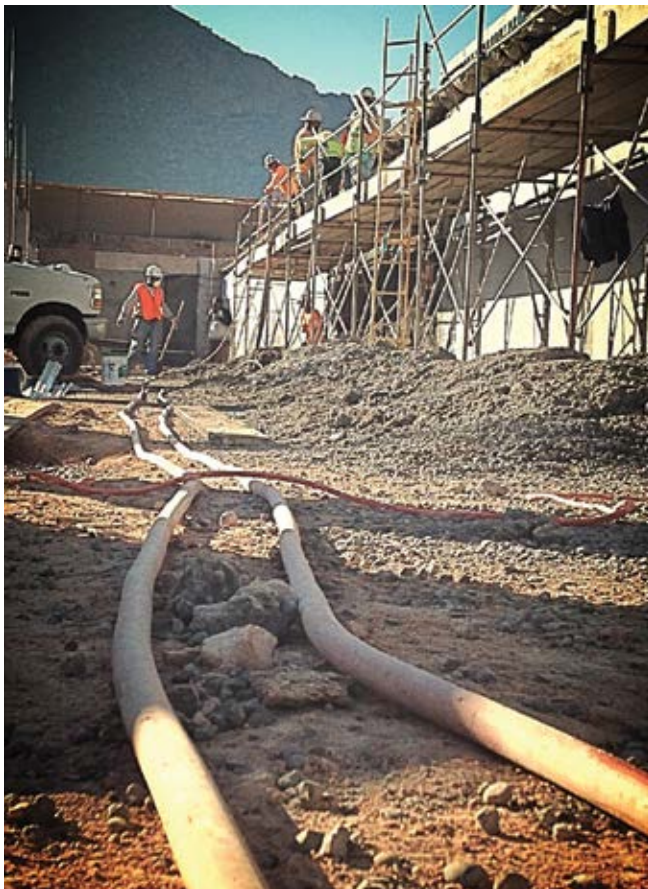
Fig 1: Longer hose lengths can lead to reduced air flow
