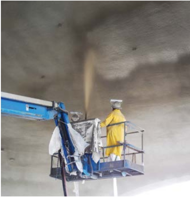
Fig. 2: Workers apply shotcrete to form the thin shell
