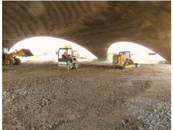
Fig. 3: Openings are made to the dome shell, which allow light to enter the completed office
