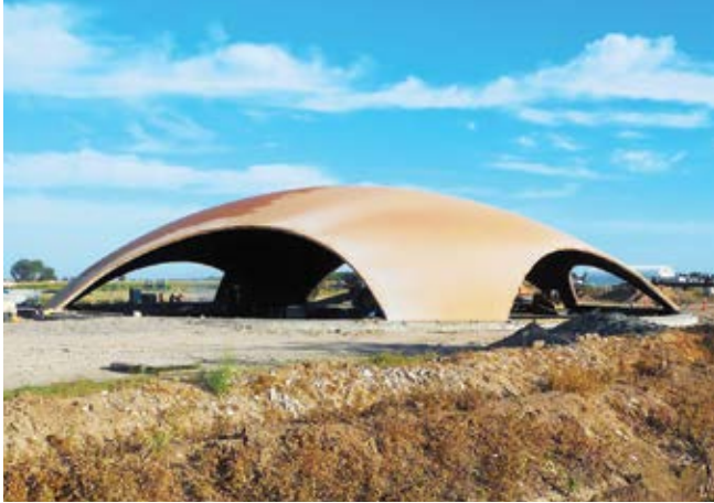
Fig. 5: A view of the dome before exterior finishes were added
