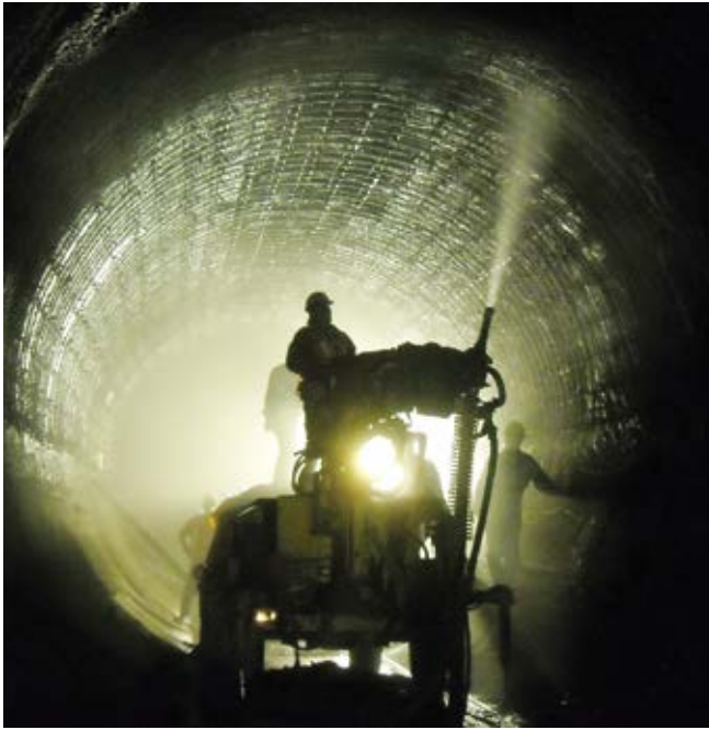
Fig. 4: Shotcreting operation
