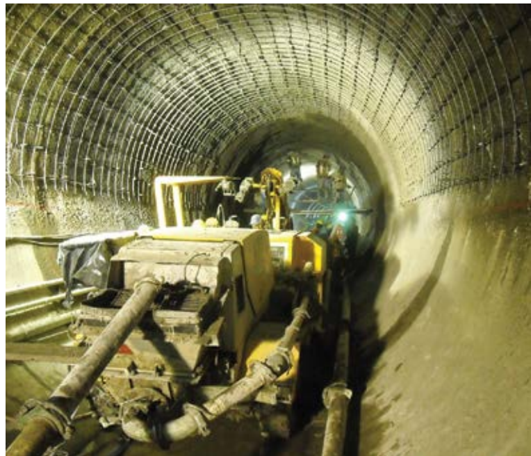
Fig. 3: Shotcrete equipment in position within the tunnel
