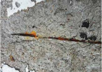
thway allowing chemical Fig. 6: Insufficient coverage over reinforcement. Reinforcement bowed outward Photo credit: Fig. 4-8 courtesy of Greg Musgrove, G & B Tile & Plaster
