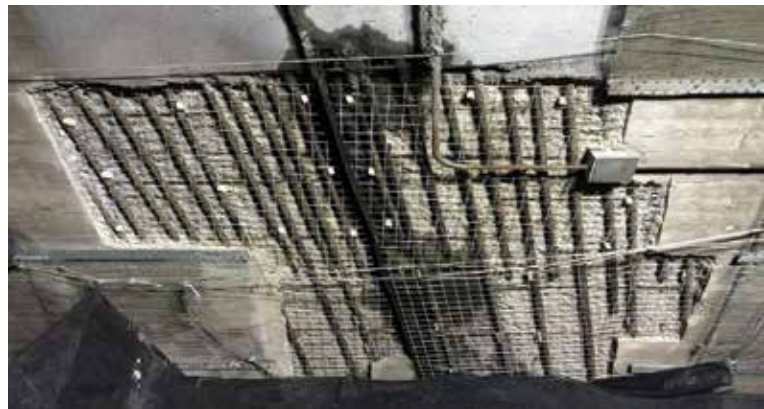
Fig.2: Anodes placed on a grid pattern
