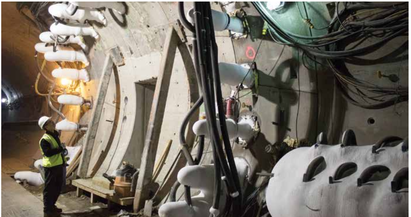
Fig. 1: Graduate student looking at the ground-freezing techniques used in the cross-passage construction on the SR99 tunnel in Seattle
