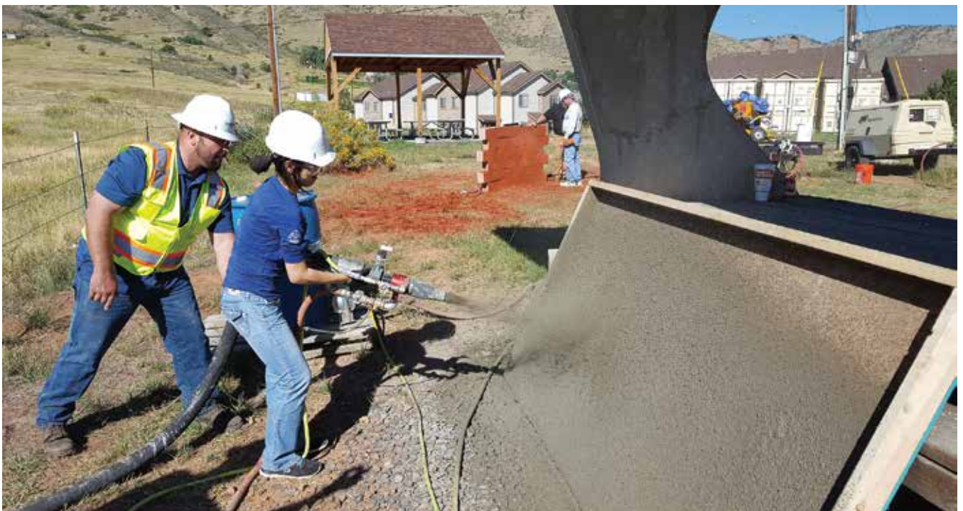
Fig. 3: Shotcrete application instruction at Shotcrete short course in September 2016
