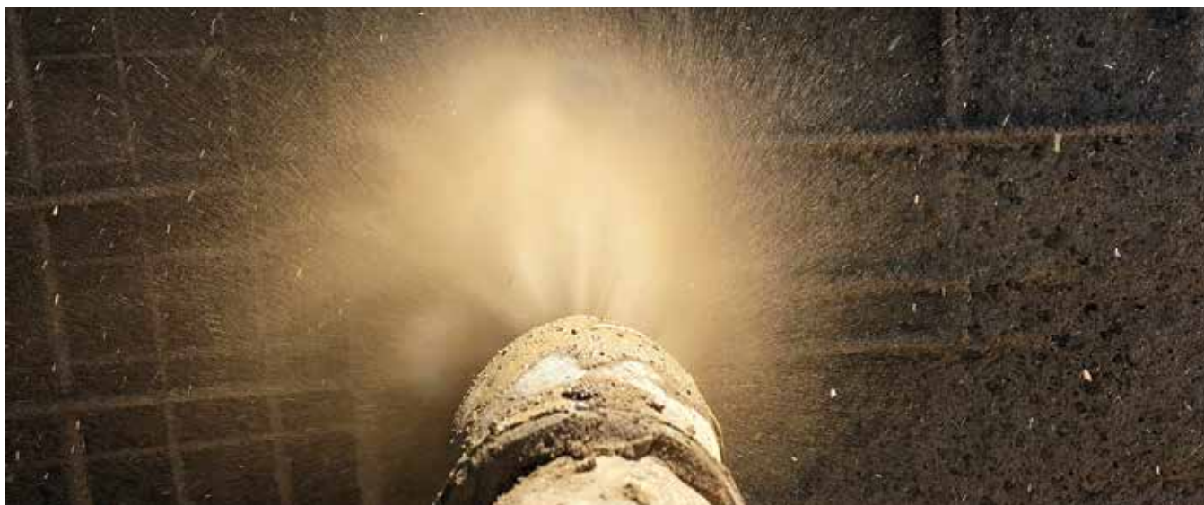
Can the skill of the nozzleman be a factor in diminishing or even eliminating rebound? The answer may surprise you
