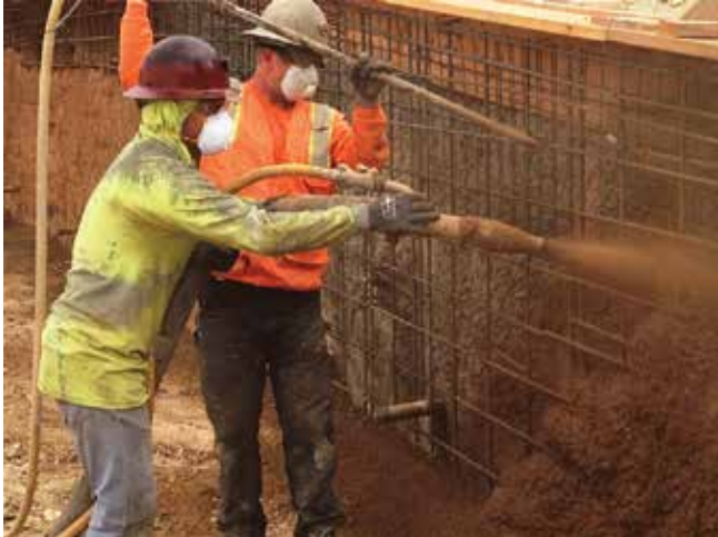
Fig. 7—The nozzleman and blow pipe operator working side by side
