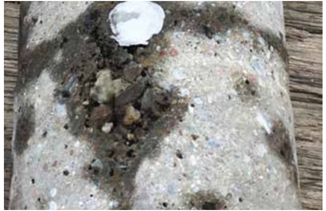
Fig. 1: Test specimen displays loose aggregates that did not fall clear of the work and became trapped behind reinforcements
