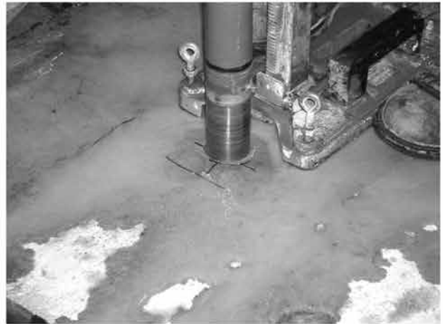
Fig. 10—Coring hole for anode.
